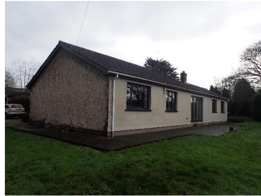
Figure 3. The property viewed from the east
