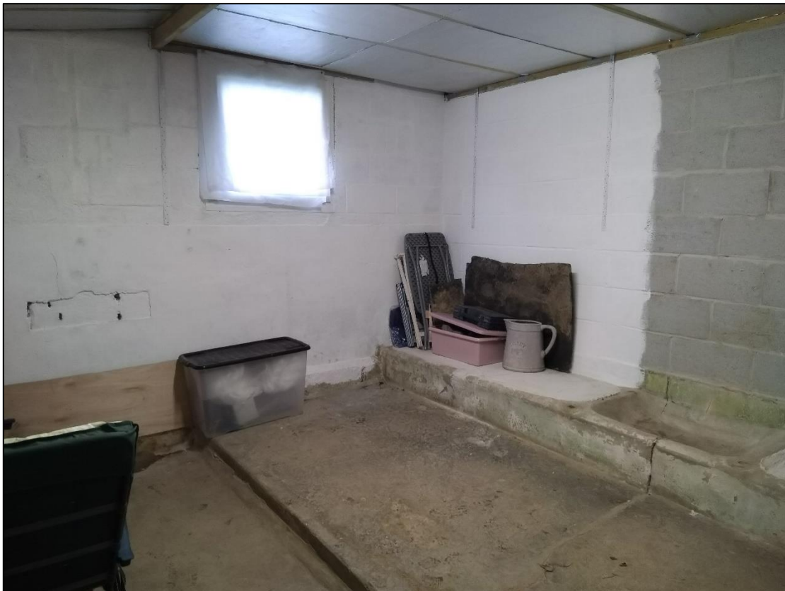
Fig 4 – Wainie's Brook Barn interior.
