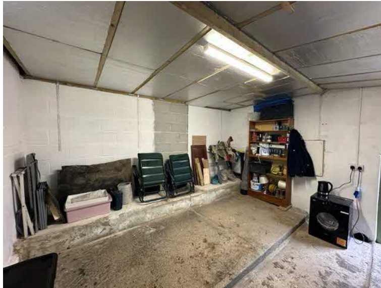
Photograph 5.0 –Pitched and vaulted roof structure from ridge beam and common rafters.
