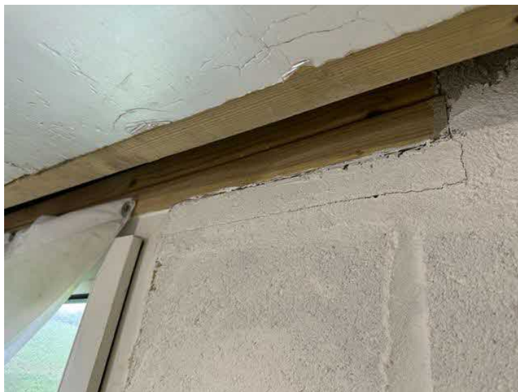
Photograph 6.0 –Timbers forming lintel over rear window opening.
