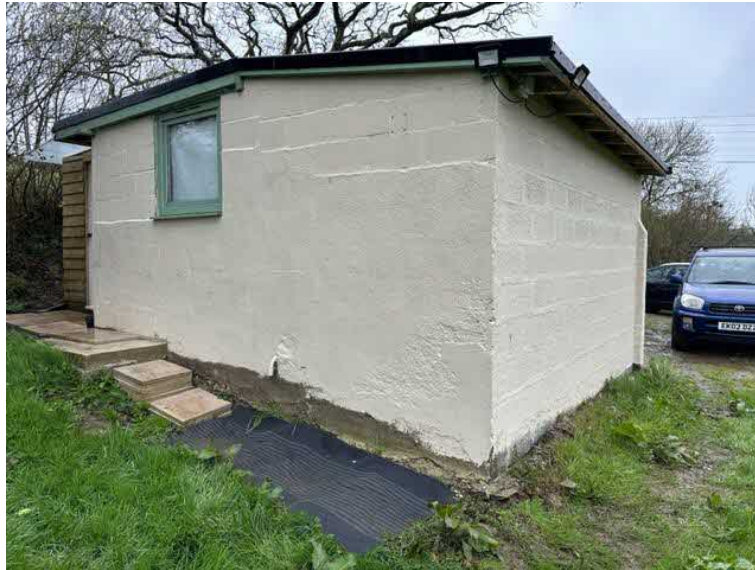
Photograph 3.0 –Southern gable wall, with increased ground levels to west end.
