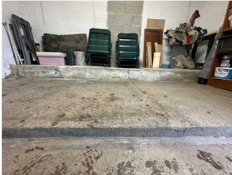
Photograph 4.0 –Internal concrete floor slab, with step (foreground) and trough beyond.
