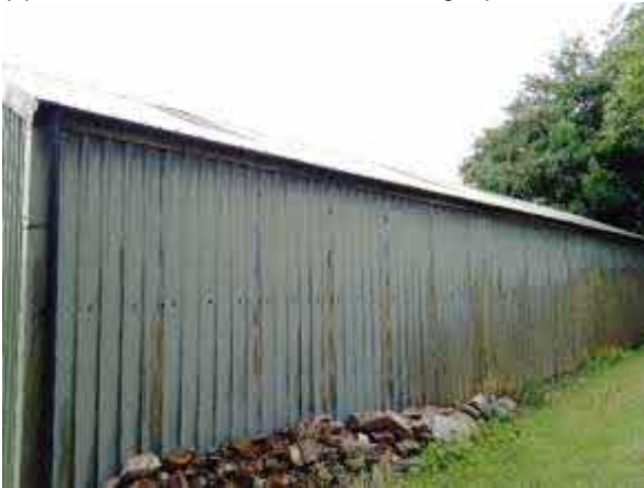
Photograph 1 – View of north side of the building.
