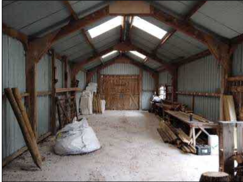
Photograph 2– Internal view of the building.
