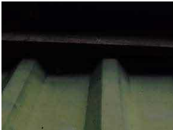
Photograph 6 – View of area of access beneath barge board.
