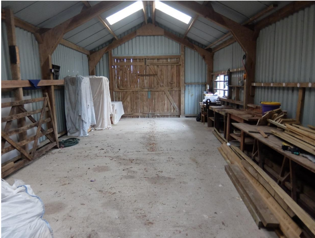
Internal view looking towards front wall
