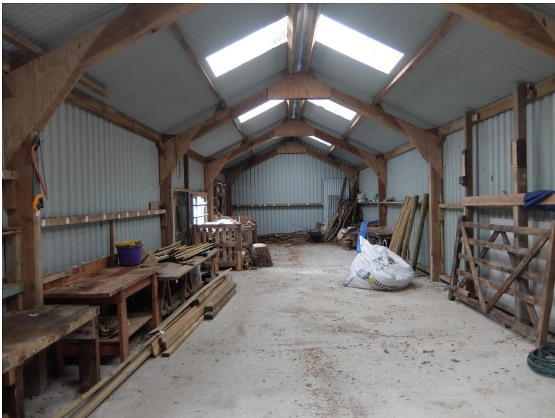
Internal view looking towards rear wall
