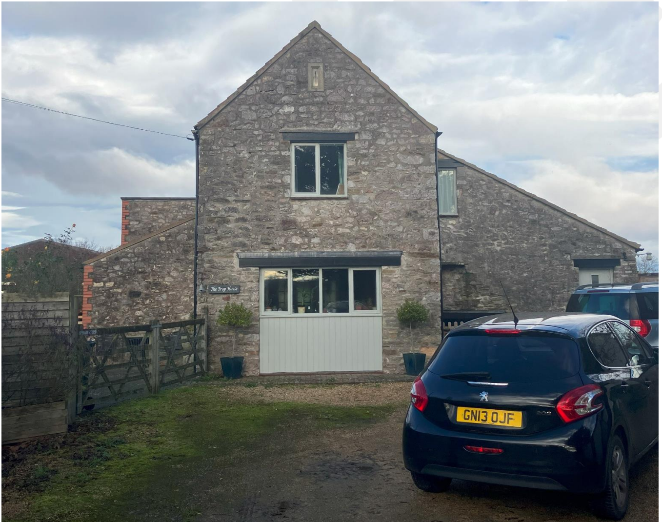
Figure 1. The Trap House Southern Elevation.
