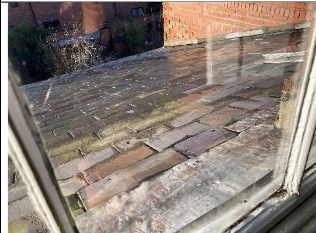
Photo 7 Single pitch over two storey section to rear
