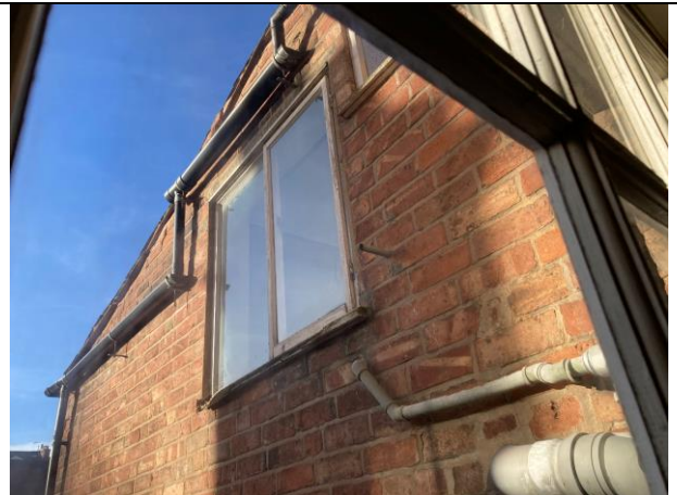
Photo 6 East verge rear (south) two storey section
