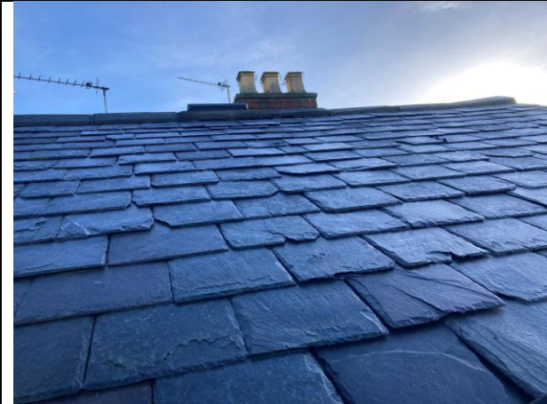
Photo 3 Main roof west pitch
