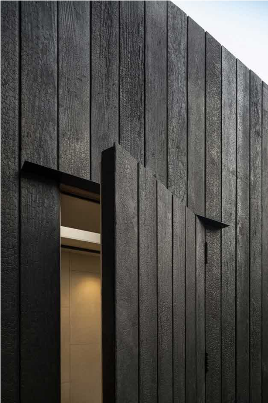
Above: Precedent image of charred timber cladding with no capping and concealed door.
