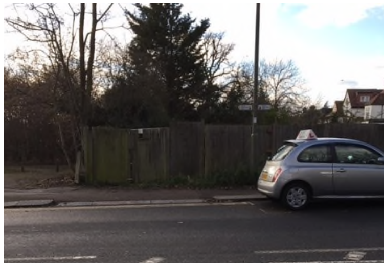
View of dropped kerb and entrance gates
