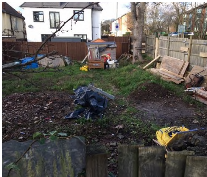
View over site from the south-east
