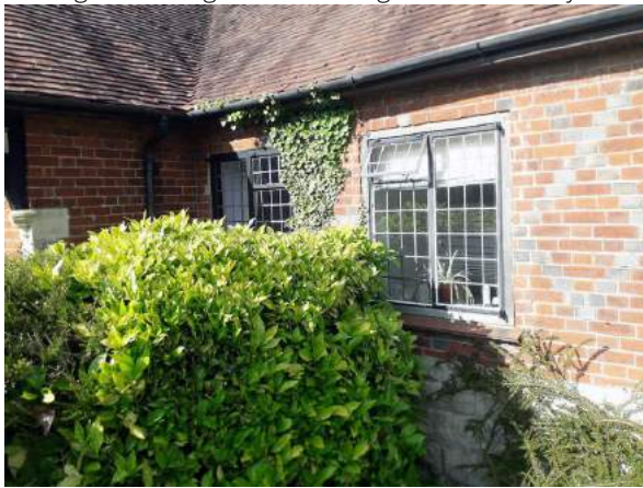
Front elevation, two windows are later additions.
