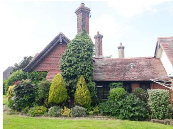
RH side elevation showing old & non-orig. extension.
