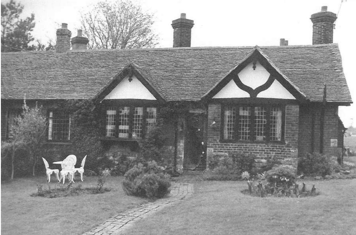
Above: Photograph of front elevation c1986, little has changed.
