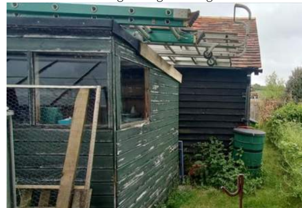
Photo showing two sheds for proposed demolition.
