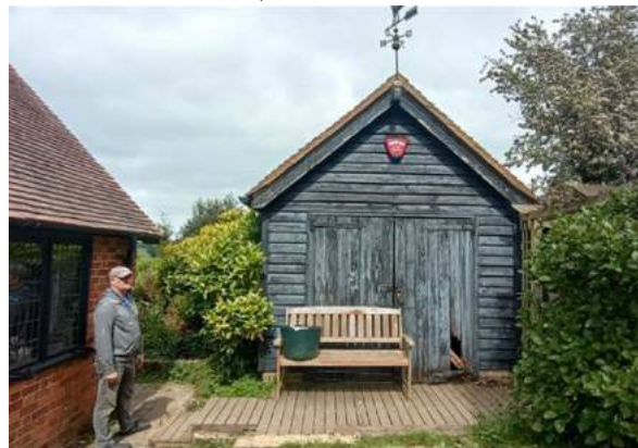
Blackened timber shed with clay tile pitched roof.
