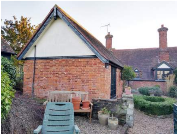
Rear elevation of later, taller addition extension.
