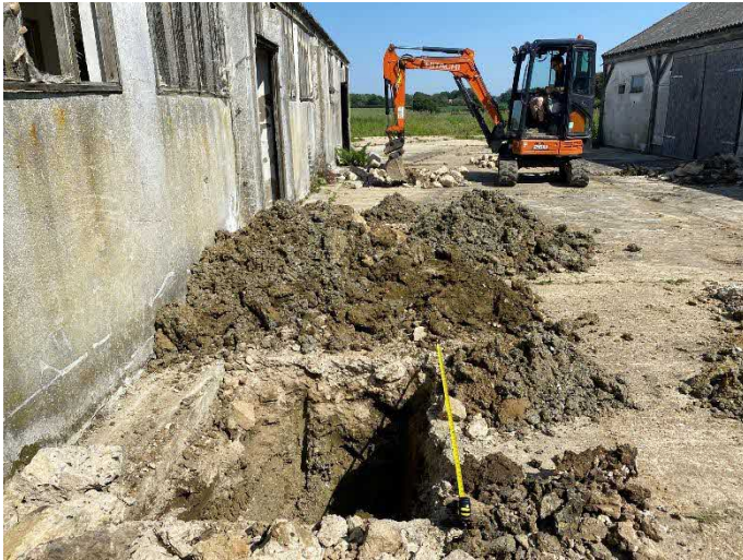
Figure 4: View of TP104.
