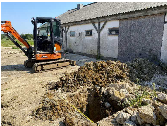
Figure 3: View of TP103.
