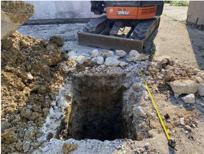
Figure 1: View of TP101.
