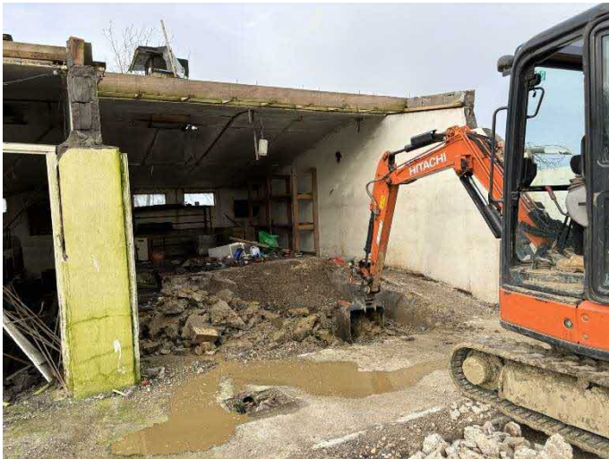
Figure 2: Excavation underway at TP201 looking north-west.
