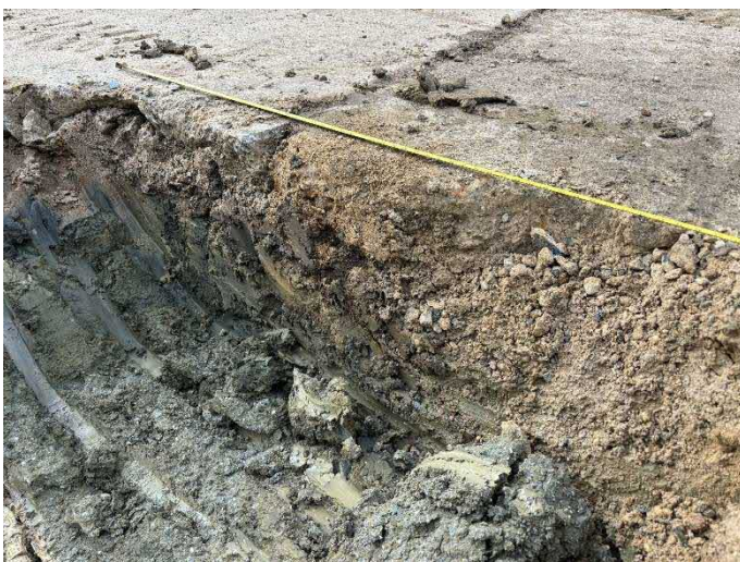
Figure 6: Encountered ground conditions within TP204.
