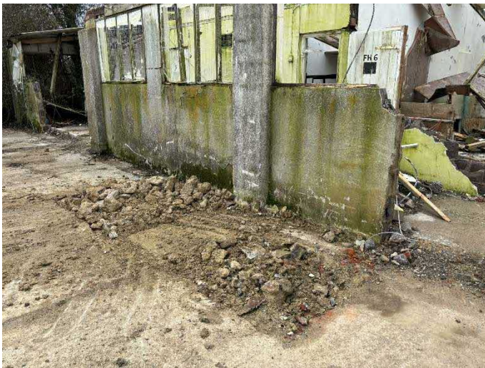
Figure 8: Backfilled position TP206.
