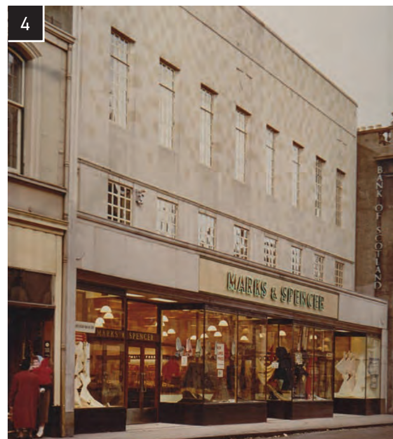
M&S store on High Street, Falkirk, c.1959
