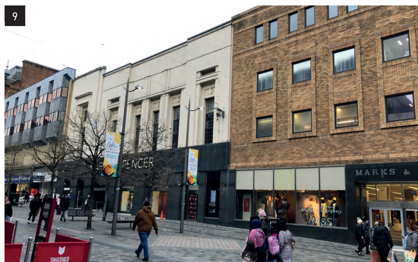
Full former M&S frontage, prior to closure of the store in April 2022, including the eastern brick-clad frontage from 1985
