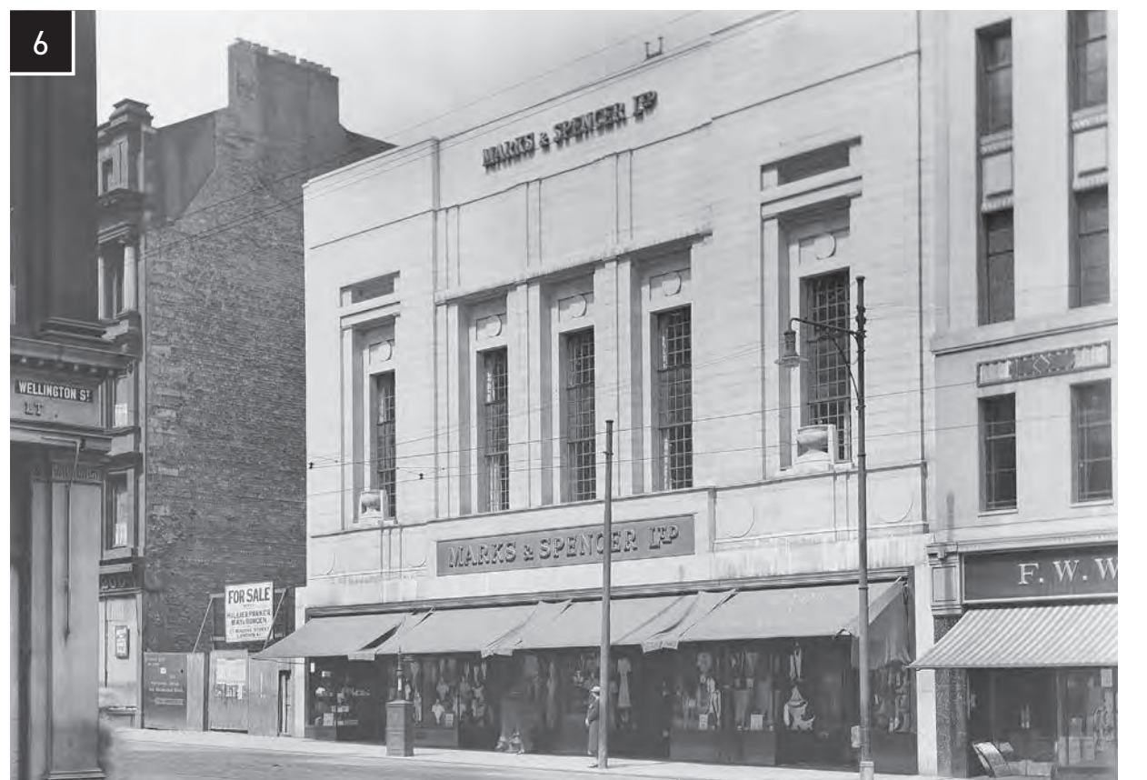
172-184 Sauchiehall Street (Marks & Spencer) in 1935 showing the building under construction. Note the plot to the immediate west which is unoccupied.
