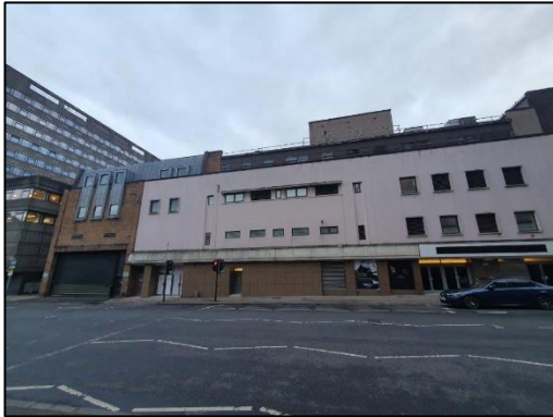
Photo 1: North aspect of the building
