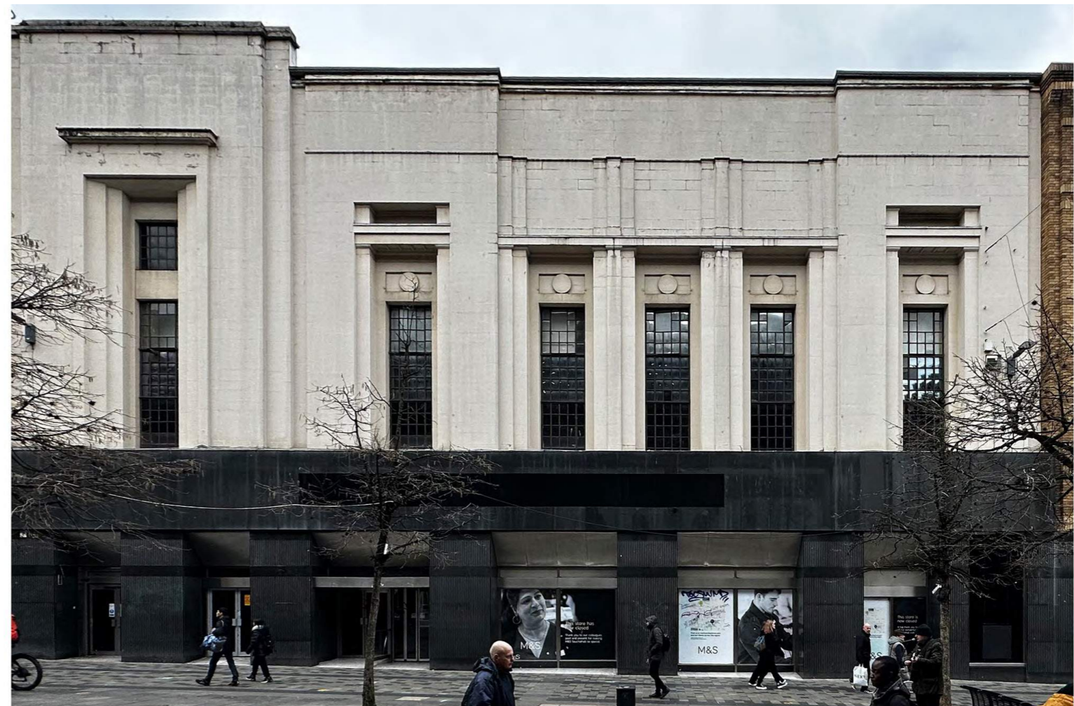
Existing Sauchiehall Street frontage
