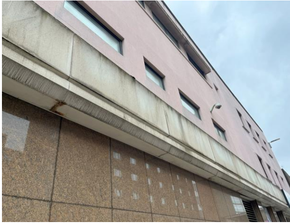
Photo 1: Outside of the building (site)
