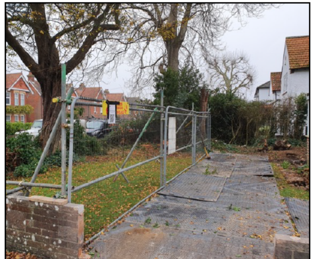
GP2: Tree protection barriers & trackmat ground protection
