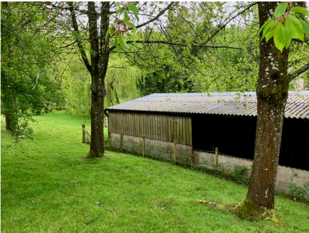
4. Rear view of The Stables
