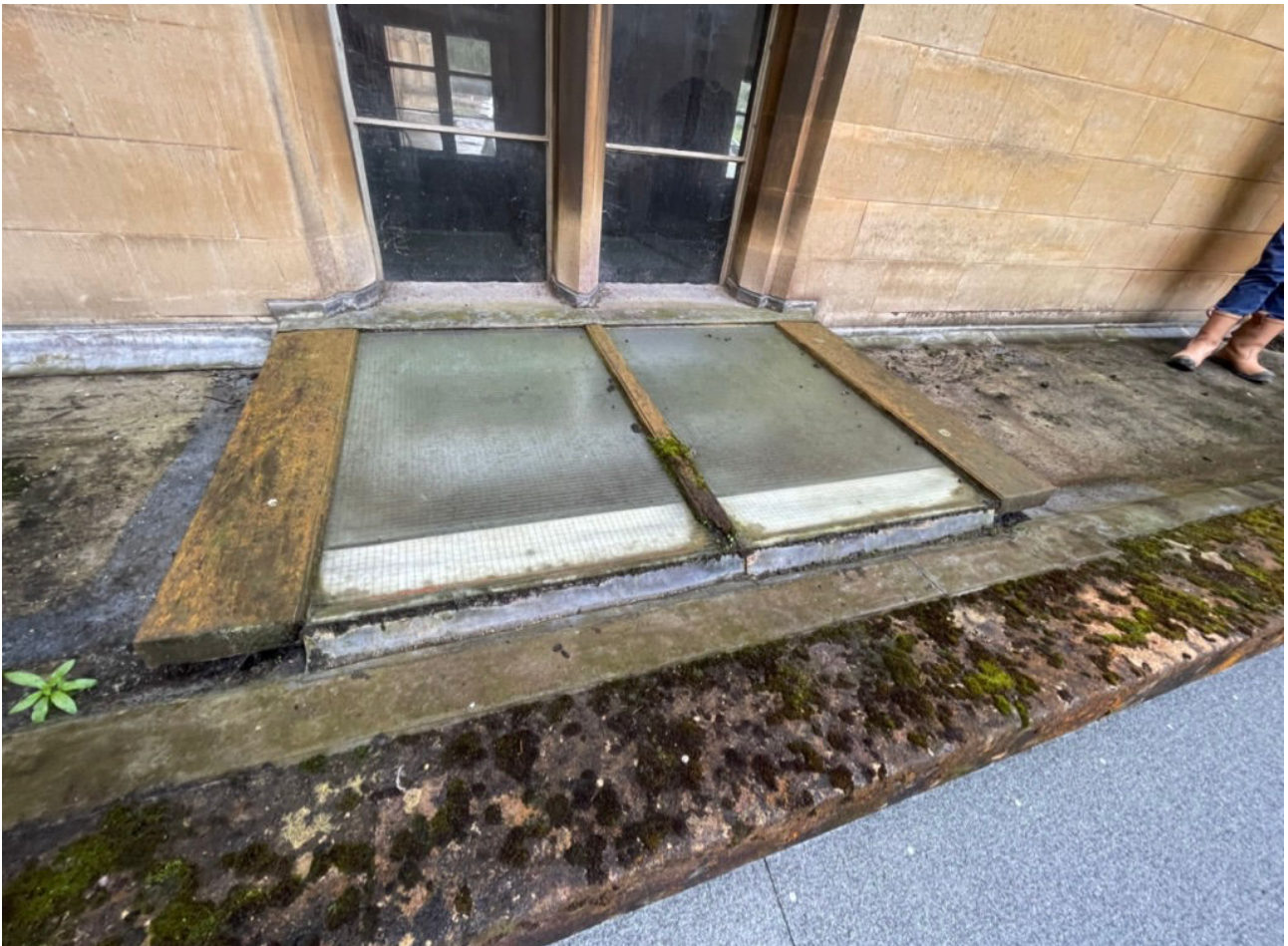
09 Looking west to rooflight r104. Modified repaired rooflight with timber glazing beads and perimeter frame. Modern Georgian wired glass and lead capped from adjacent window we02. Note very narrow perimeter gutter to eastern edge of r104, subsequently lined with lead flashing.
