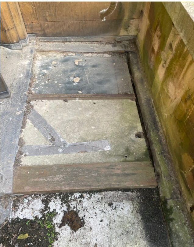
13-14 Looking north to rooflight r105. Roof is very constrained in this area with very narrow, c.60mm wide deep gutter leading to outfall at north end of roof – through outlet reduced to 40ø as it passes through wall to hopper. Proposal is to diamond core drill to allow provision of 100ø pipe through wall.
