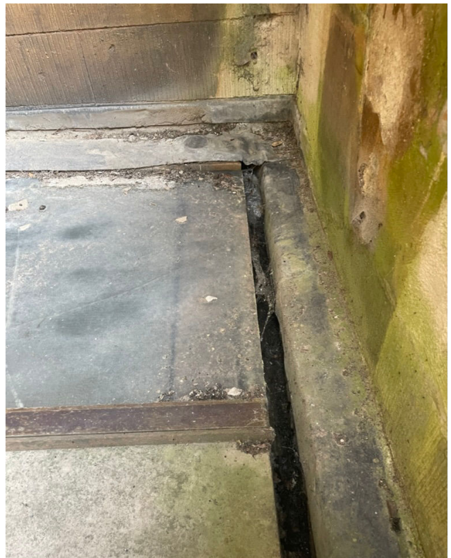
13-14 Looking north to rooflight r105. Roof is very constrained in this area with very narrow, c.60mm wide deep gutter leading to outfall at north end of roof – through outlet reduced to 40ø as it passes through wall to hopper. Proposal is to diamond core drill to allow provision of 100ø pipe through wall.
