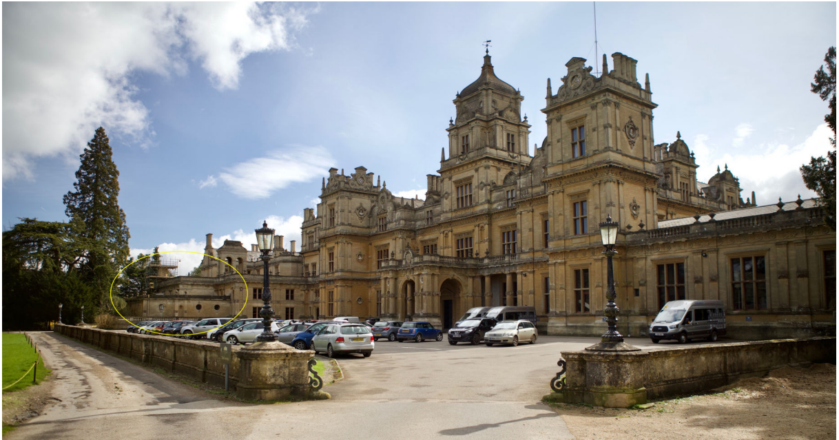
01 Westonbirt House general view of the north elevation and forecourt, with symmetrical central range, five-storey tower with ogee roof and corner turrets. The similarities with Wollaton Hall in Nottingham are quite striking. Note: location of proposed works to the north east office range rooflights r101- r105 inclusive (circled in yellow).
