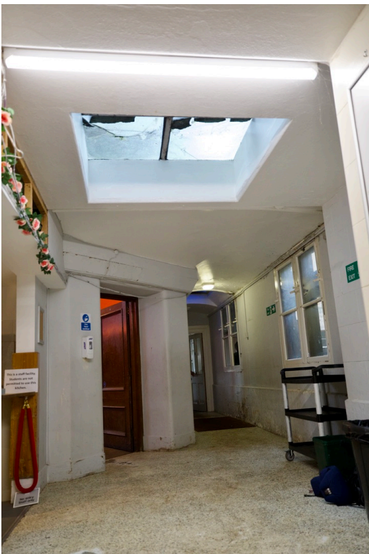
17-18 Looking north below rooflight r102. Rooflight is at south end of the access corridor to the service wing, adjacent to the entrance to the refectory. Existing rooflight suffers repeated water penetration and algal growth following damage [cracks] to 2no replacement Georgian wired glass lights.
