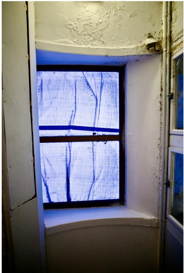
21-22 Looking north towards and below rooflight r104. Rooflight towards south end of the west corridor. Repeated water penetration throughout this area, with mould and algal growth to trimmed roof structure. Mat laid below rooflight to collect drips and reduce trip hazard in corridors [nb: rooflight covered with blue tarpaulin to prevent severe water ingress since photographs 09-11 taken externally].
