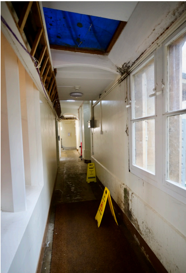
24-25 Looking north and south from r105. With evidence of water penetration throughout north end of corridor.
