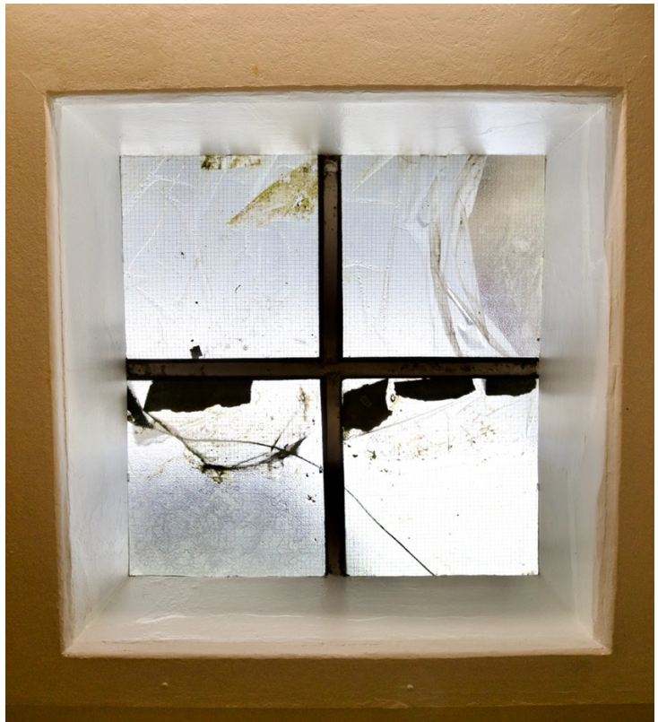
17-18 Looking north below rooflight r102. Rooflight is at south end of the access corridor to the service wing, adjacent to the entrance to the refectory. Existing rooflight suffers repeated water penetration and algal growth following damage [cracks] to 2no replacement Georgian wired glass lights.
