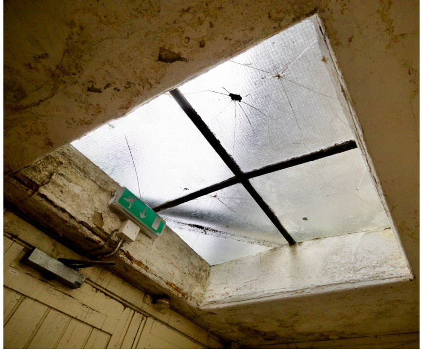
19-20 Looking north below rooflight r103. Rooflight is above the entrance porch to the south west corner of the courtyard. Significant repeated water penetration to all edges of roof and through glazing bars. Damaged to Georgian wired glass.
