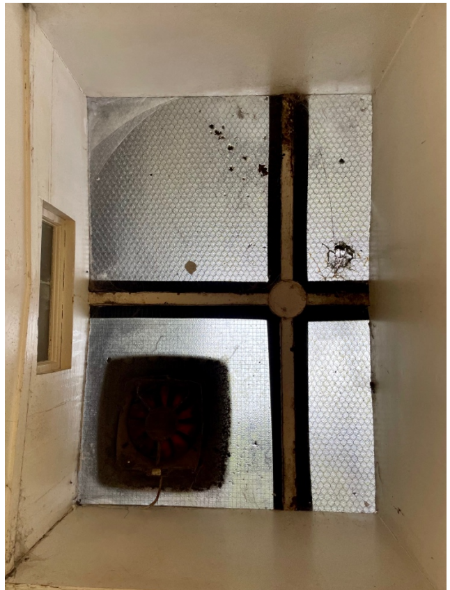
15-16 Looking north below rooflight r101. Rooflight only partly visible within male students wc, having been obscured by later internal blockwork wall to east. Note water penetration to sides of lantern, redundant extract fan and variety of replacement Georgian wired glass (and damage). Glazing bars appear wider and more significant as a result of flashband repairs externally and electrical conduit installation internally.
