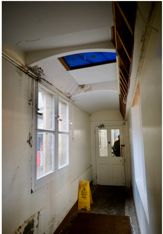
24-25 Looking north and south from r105. With evidence of water penetration throughout north end of corridor.
