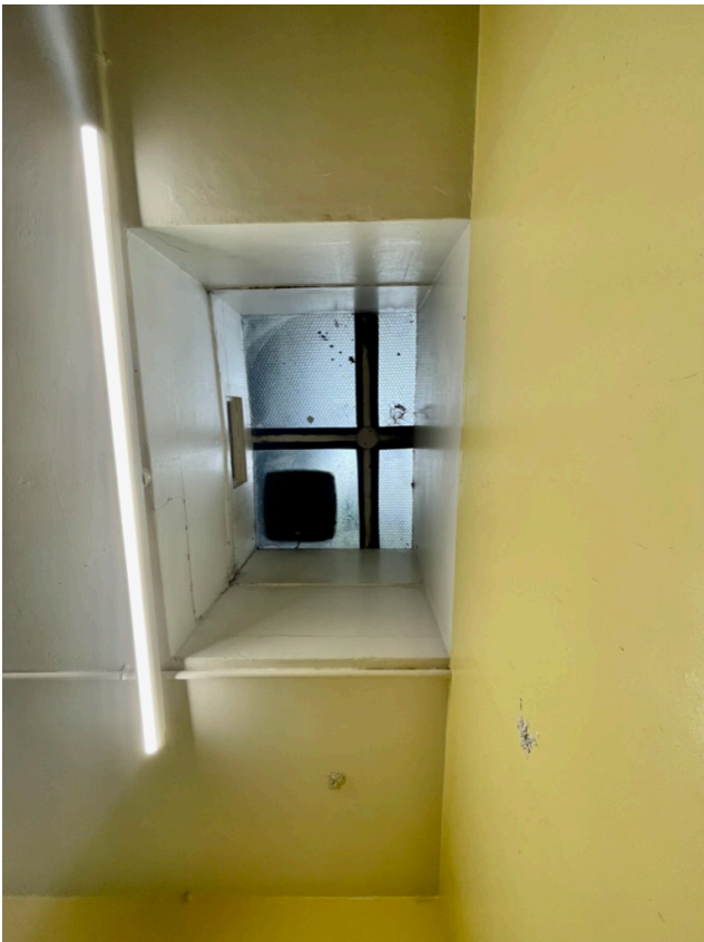
15-16 Looking north below rooflight r101. Rooflight only partly visible within male students wc, having been obscured by later internal blockwork wall to east. Note water penetration to sides of lantern, redundant extract fan and variety of replacement Georgian wired glass (and damage). Glazing bars appear wider and more significant as a result of flashband repairs externally and electrical conduit installation internally.
