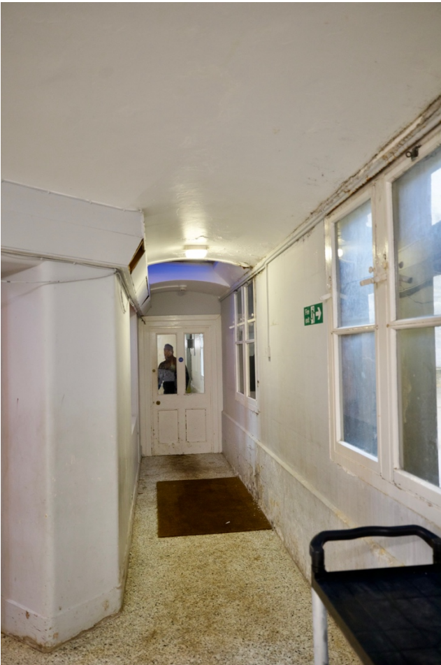
21-22 Looking north towards and below rooflight r104. Rooflight towards south end of the west corridor. Repeated water penetration throughout this area, with mould and algal growth to trimmed roof structure. Mat laid below rooflight to collect drips and reduce trip hazard in corridors [nb: rooflight covered with blue tarpaulin to prevent severe water ingress since photographs 09-11 taken externally].
