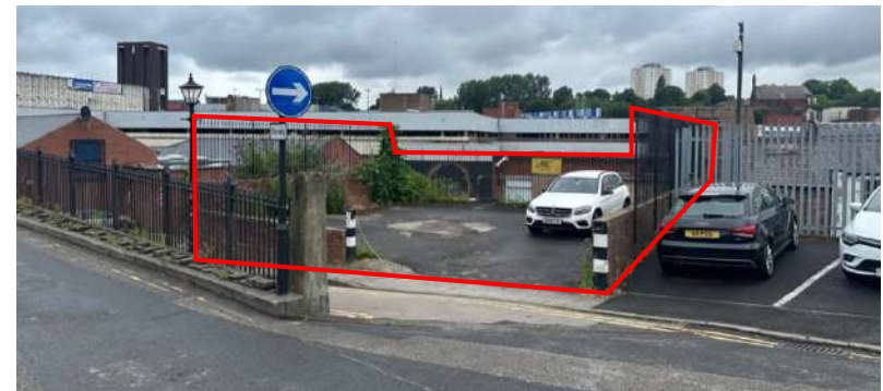
Figures 4.12 & 4.13: The Application Site from High Bank Side (2023)
