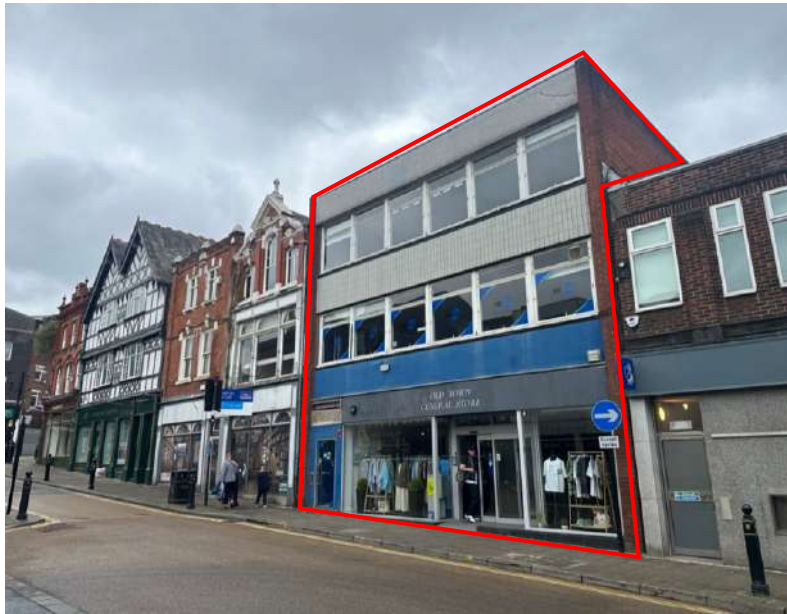
Figure 4.9: The Application Site from Great Underbank (2023)
