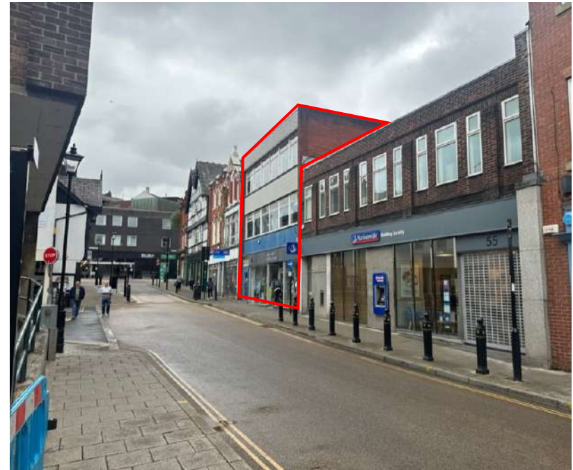
Figure 4.10: The Application Site from Great Underbank (2023)
