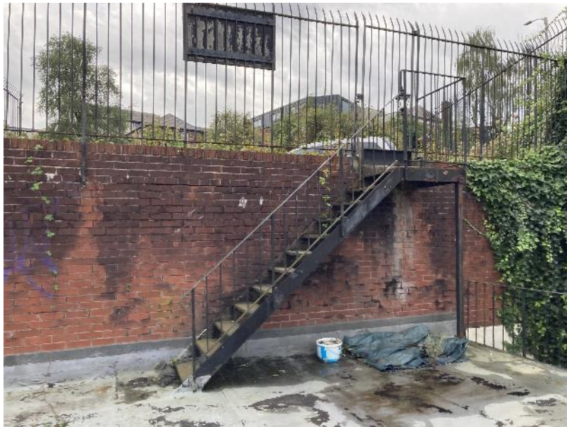
PLATE 8 SHOWING RED BRICK RETAINING WALL
