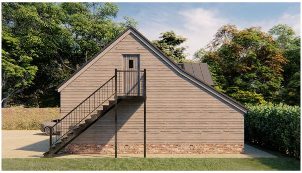
The material palette has been altered to comprise of a brick plinth and timber boarding to external elevations. The roof will be seamed aluminium or similar.
