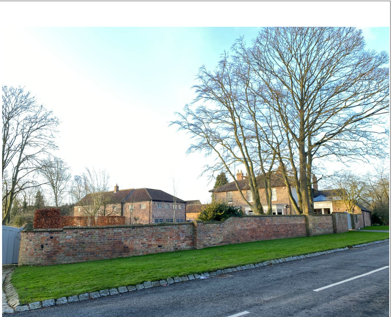
Fig C – Use of lantern rooflight in context with older property.
