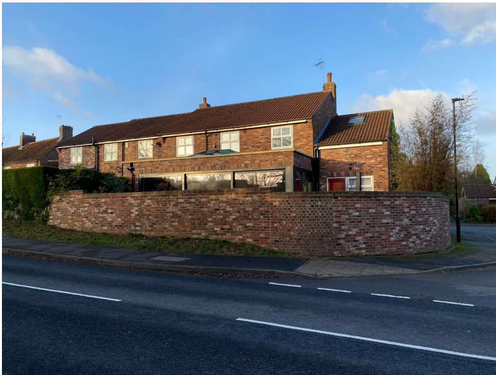
Fig A - Lantern rooflight partially concealed behind parapet wall and does not dominate overall appearance.
