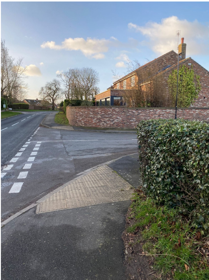
Fig B - Same extension / lantern viewed from farther away, lantern barely visible.
