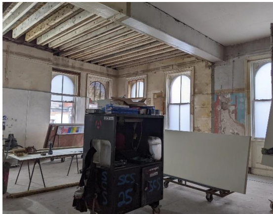
Photo 3: windows obscured by former kitchen
