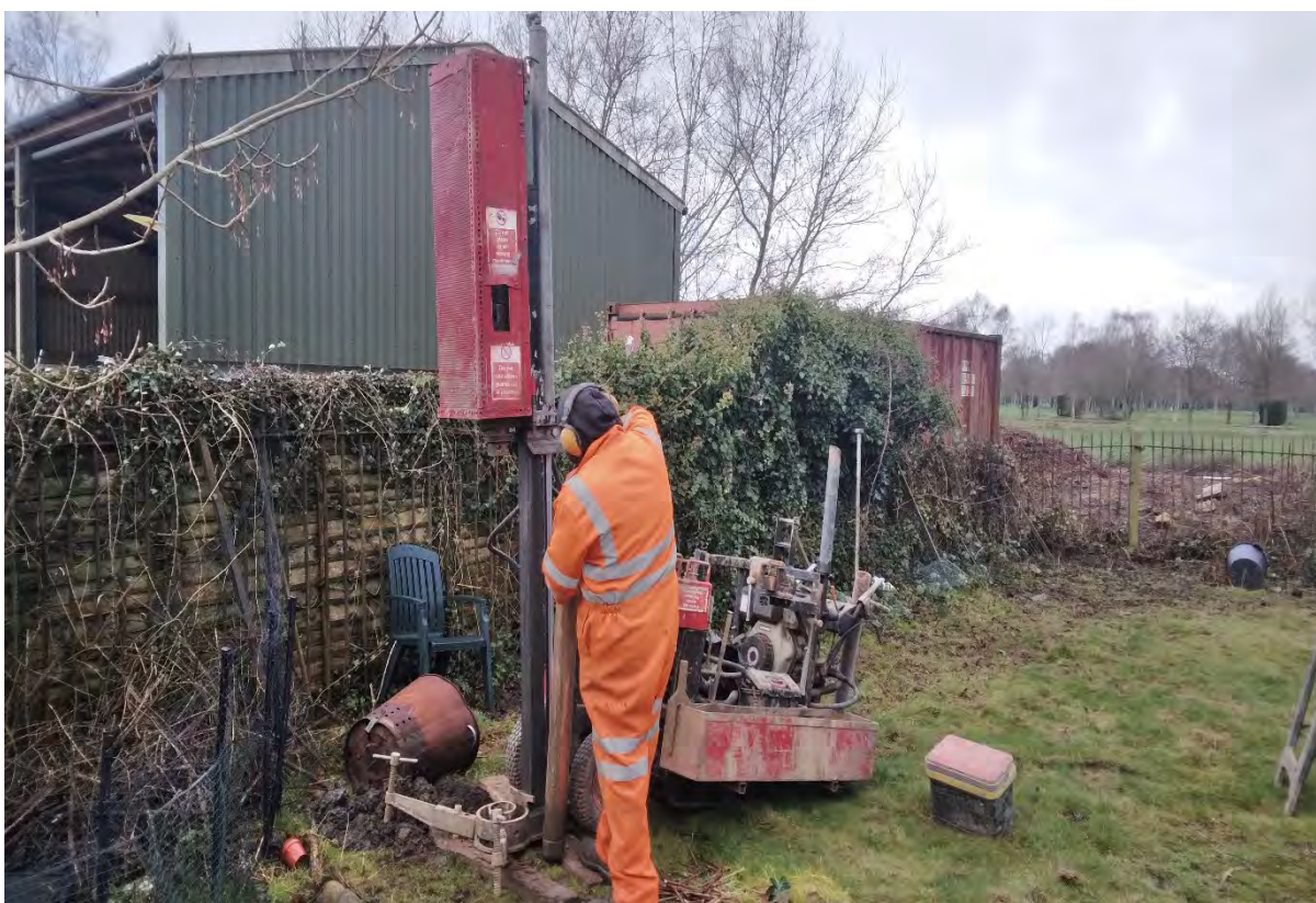
View northwest towards BH01 during drilling.
