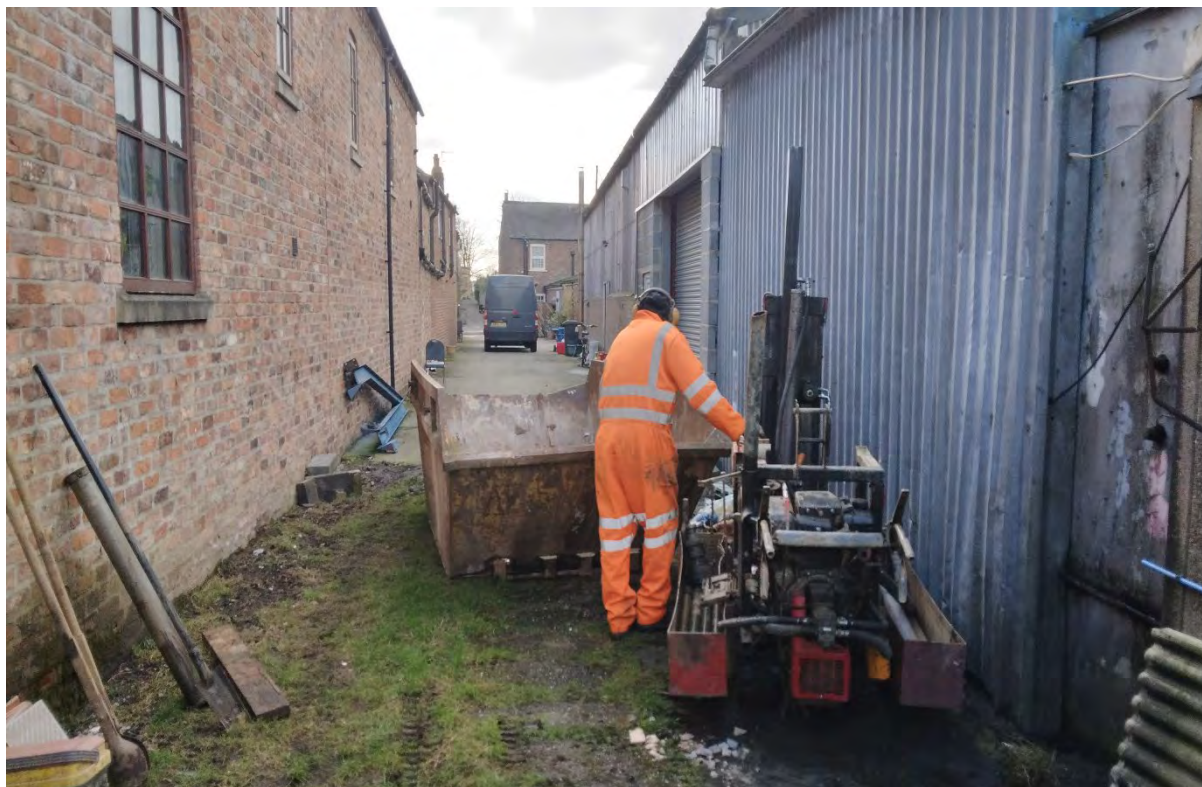
View southeast through the site towards BH03 during drilling.
