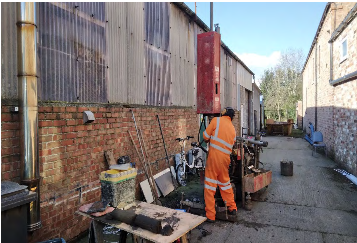
View northwest towards BH04 during drilling.
