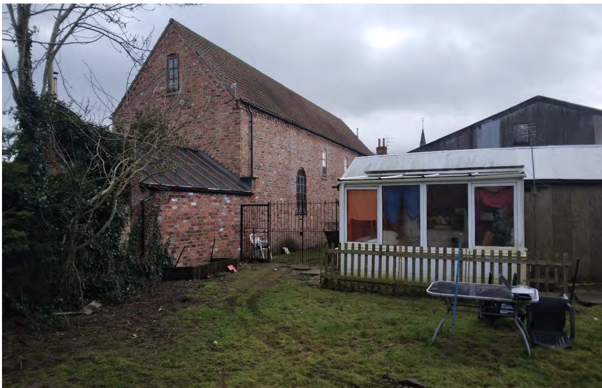
View southeast across the northern portion of the site.
