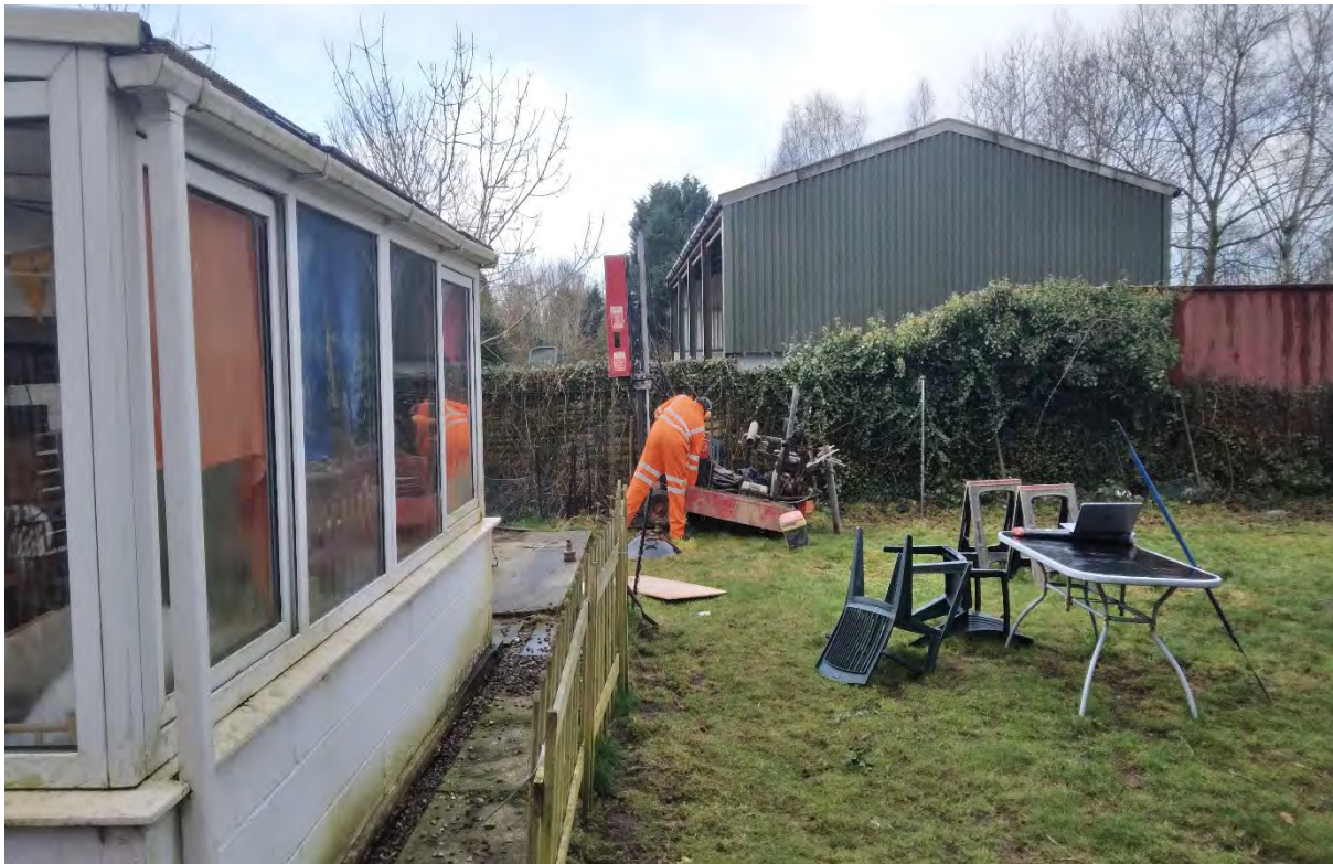
View west across the northern portion of the site towards BH01.
