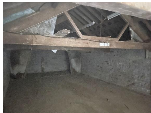
Plate 6: Barn – Interior (Upper-floor)
