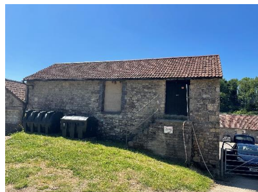
Plate 2: Barn (Northern Aspect)
