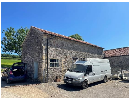
Plate 1: Barn (Southern Aspect)
