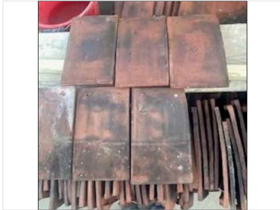
CLAY PEG TILES TO MATCH EXISTING
