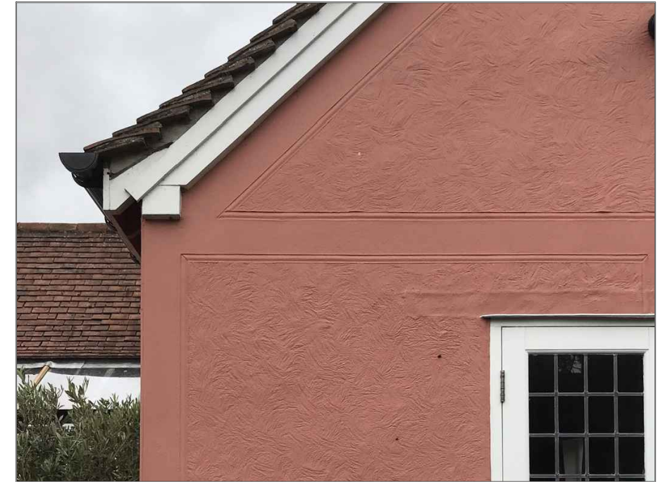
LIME RENDERED WALLS WITH PARGETING, PAINTED IN SUFFOLK PINK TO MATCH EXISTING
