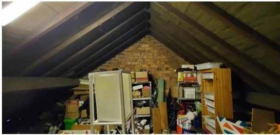
5 Internal view of loft
