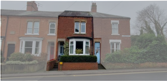
1 Front – north west aspect
