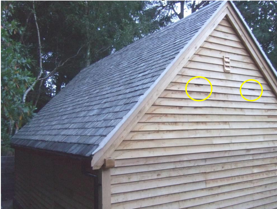
Figure 4 – showing the positioning of the pipistrelle roost boxes in the proposed bat barn and the bat access louvers. The same detail in each gable
