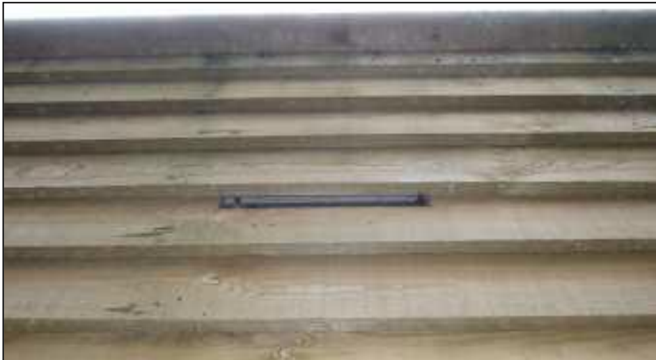
Figure 4c: example photograph of the Batbox when set behind oak panelling, with the slot provided for access.
