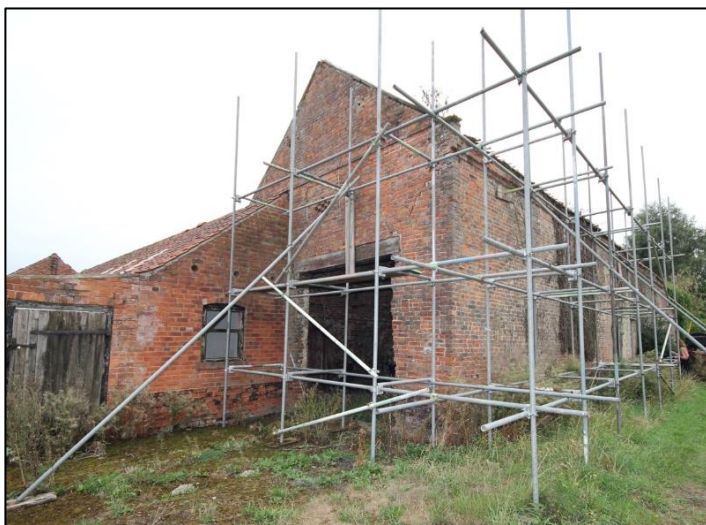
Plate 26: View towards east elevation of Building B.
