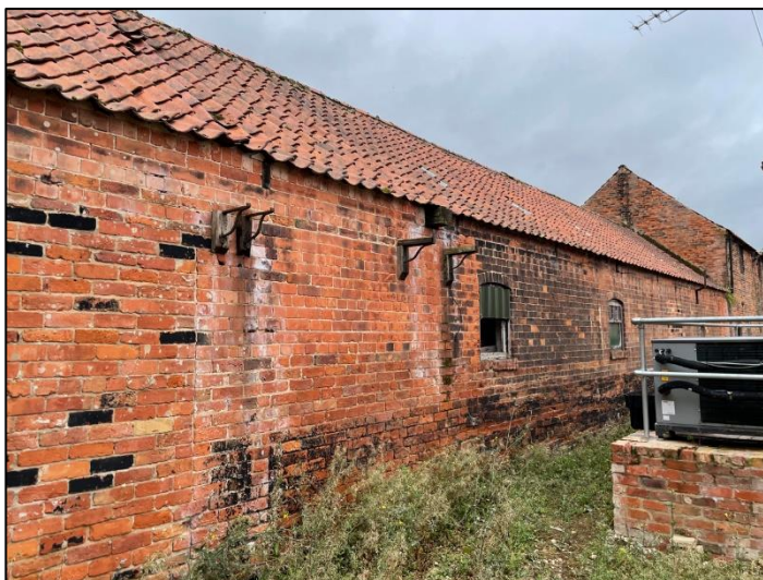
Plate 32: View towards west elevation of Building C looking south-east.
