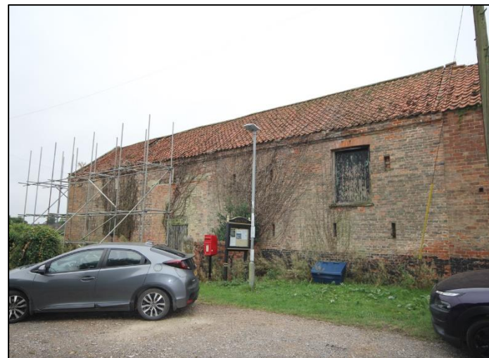
Plate 24: View towards north elevation of Building B.
