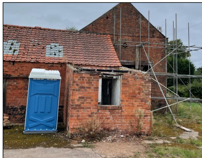
Plate 36: View towards east elevation of abutting wing to Building C.
