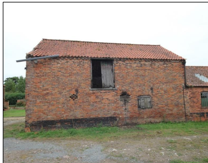
Plate 46: View towards east elevation of Building D.
