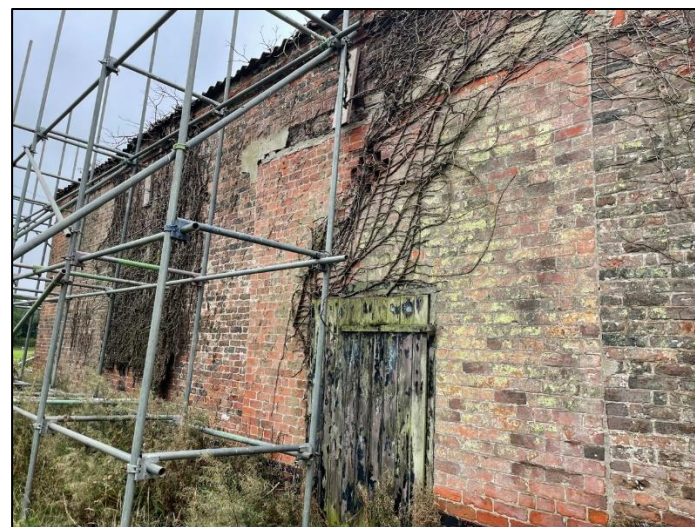
Plate 25: Brick infilled threshing door to north elevation of Building B.
