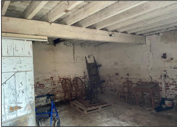
Plate 17: Internal view of northern wing of Building A looking north.
