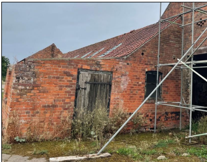
Plate 37: View towards north elevation of abutting wing to Building C.
