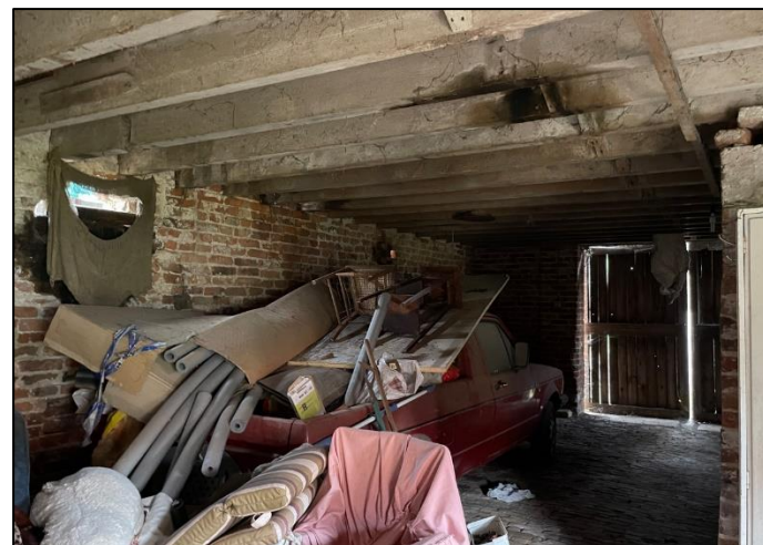
Plate 48: Internal view of ground floor to Building D looking south-east.
