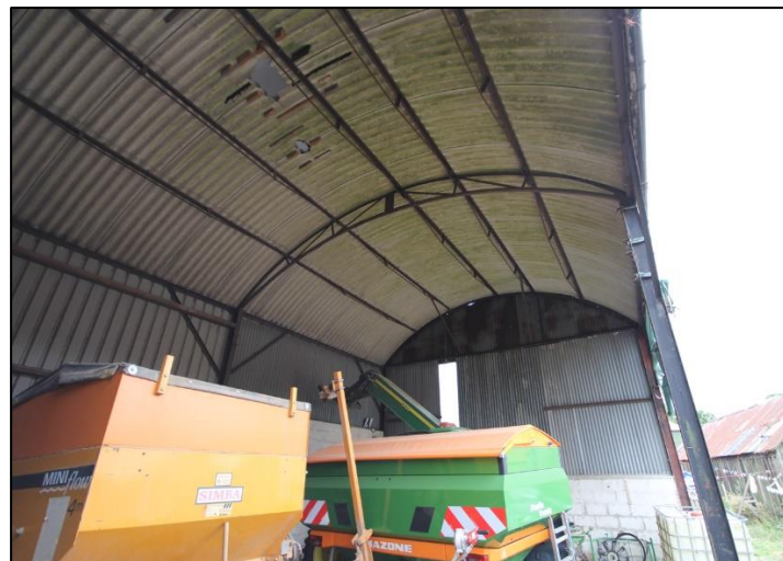
Plate 54: Internal view of Dutch Barn looking south.
