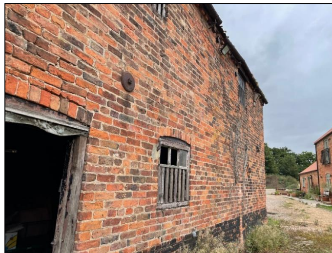
Plate 45: View towards west elevation of Building D.
