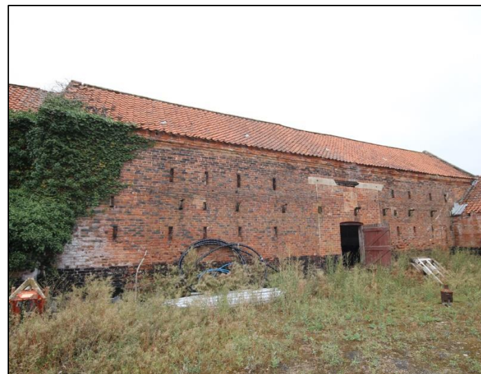
Plate 27: View towards south elevation of Building B.
