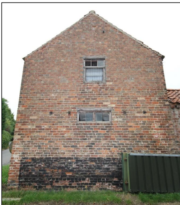
Plate 15: View towards west elevation of northern wing to Building A.
