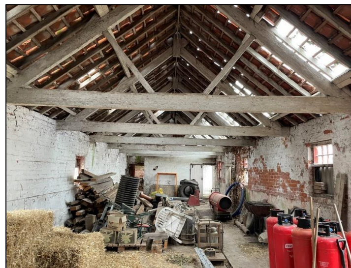
Plate 38: Internal view of Building C looking north.
