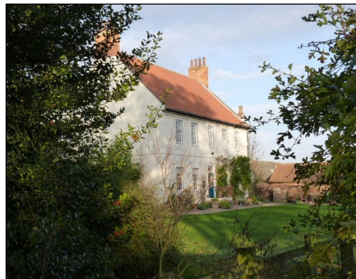
Plate 63: View towards principal north elevation of The Grange.
