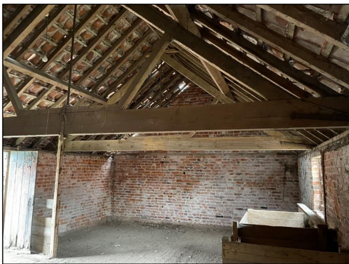
Plate 50: Internal view of first floor to Building D looking south.
