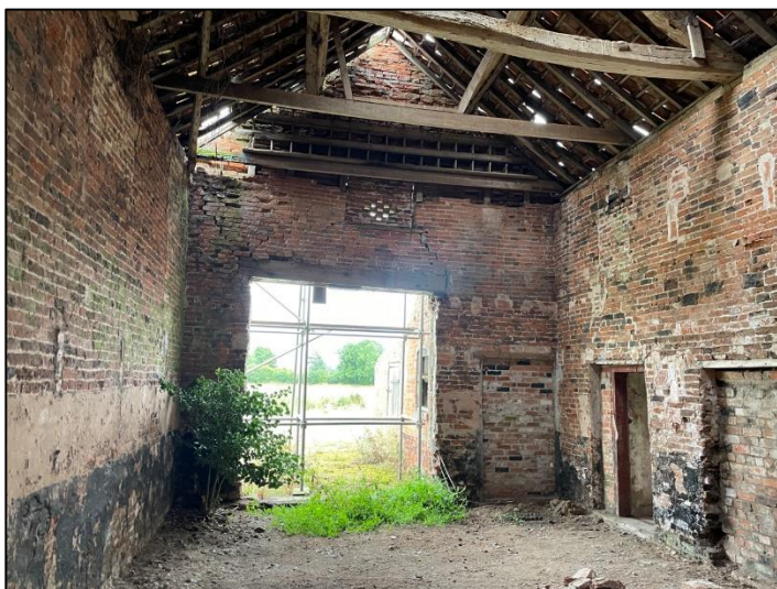
Plate 28: Internal view of Building B looking east.
