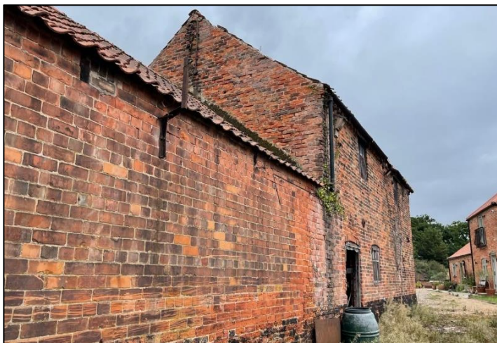
Plate 44: View towards west elevation of Building D.
