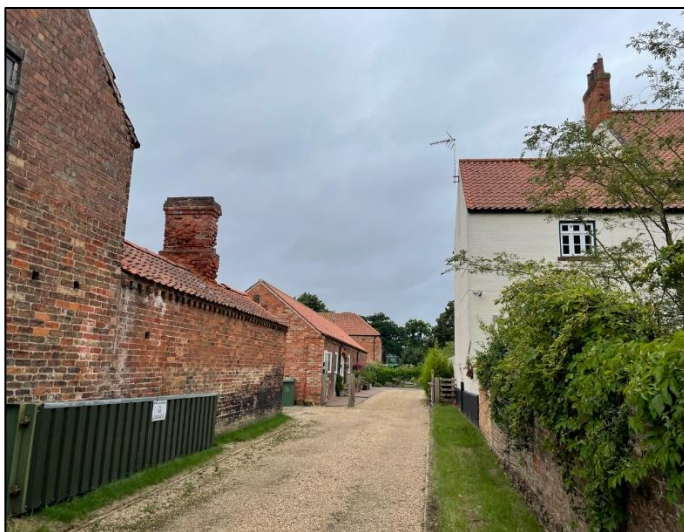
Plate 64: View looking south along the intervening access track between the Site (left) and The Grange (right).
