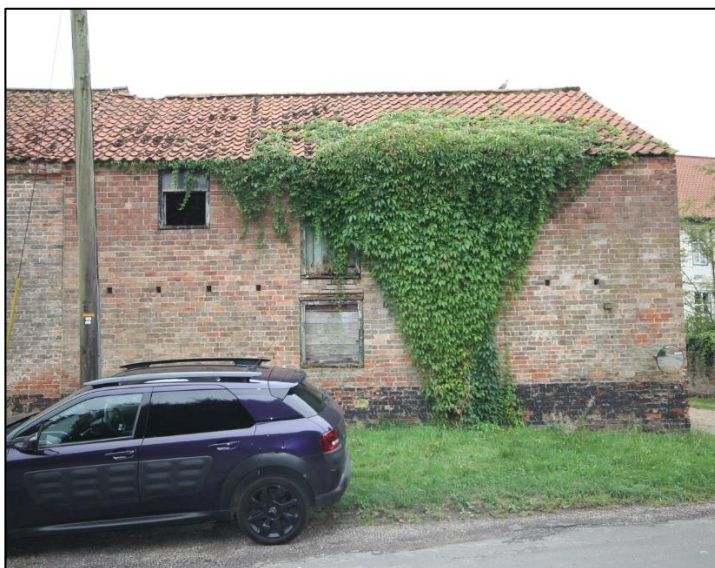
Plate 13: View towards north elevation of northern wing to Building A.
