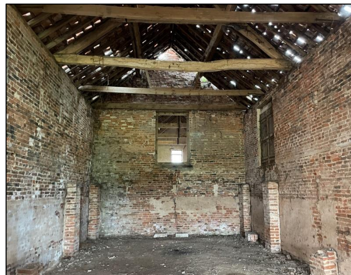
Plate 29: Internal view of Building B looking west.
