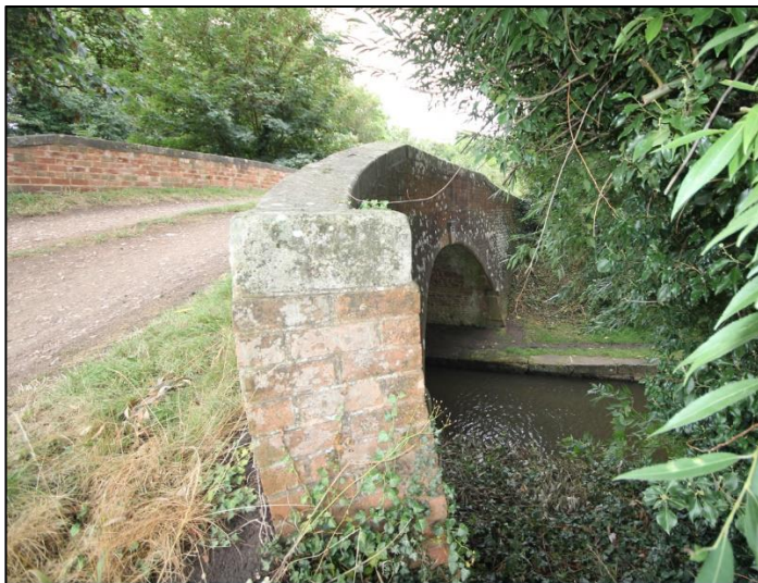
Plate 70: Wiseton Top Bridge viewed from the south.
