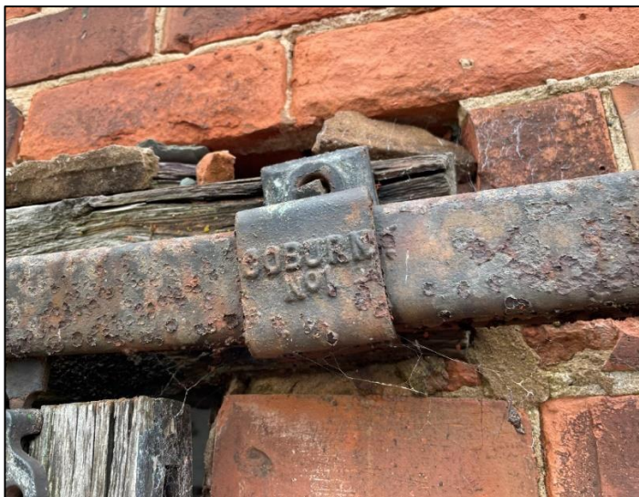
Plate 35: Maker's mark to iron door sliding rail.
