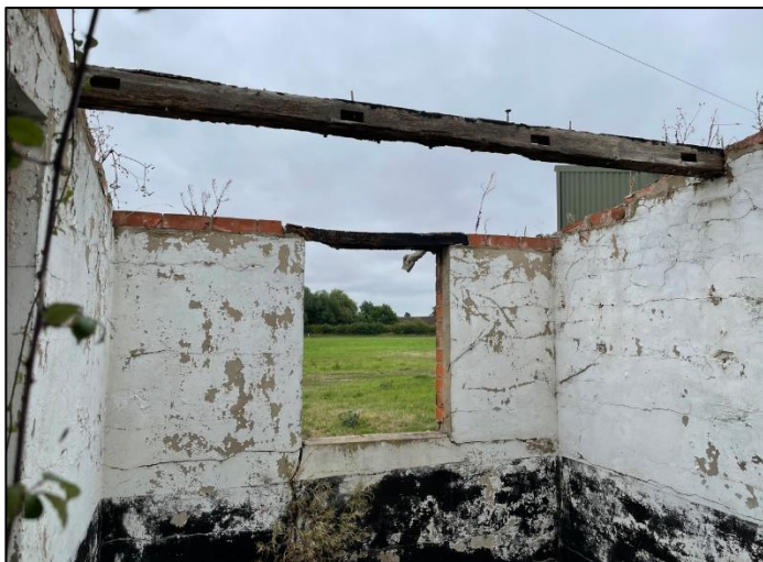
Plate 42: Internal view of abutting wing to Building C looking east.
