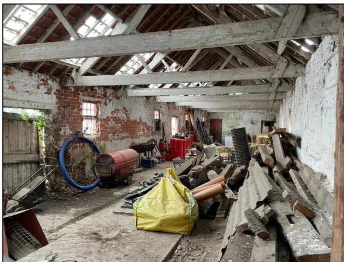
Plate 39: Internal view of Building C looking south.
