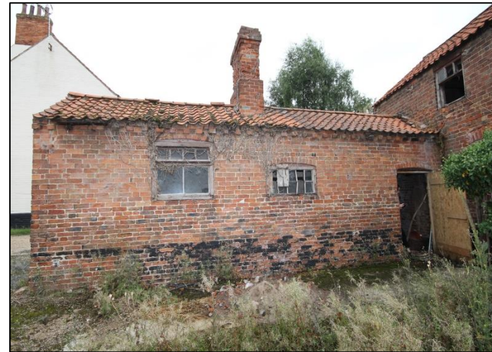
Plate 18: View towards east elevation of western wing to Building A.
