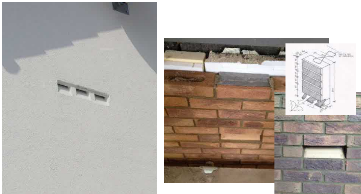
Figure 4: Examples of bat tubes fitted within the brickwork of an exterior wall
