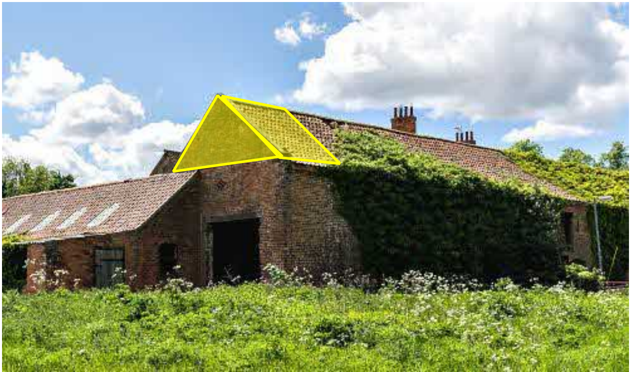
Figure 2: The position of the proposed bat attic within the roof void of the threshing barn.
