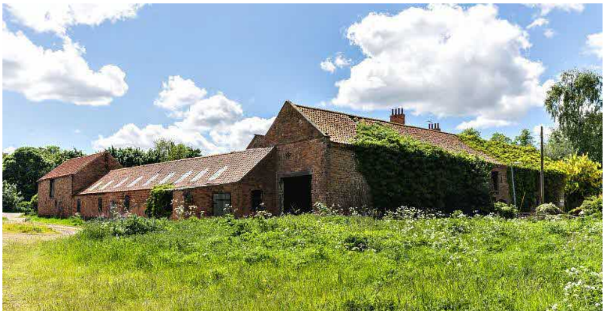
Photograph 2: Buildings A and B to the right and C and D to the left, taken from the north-east.
