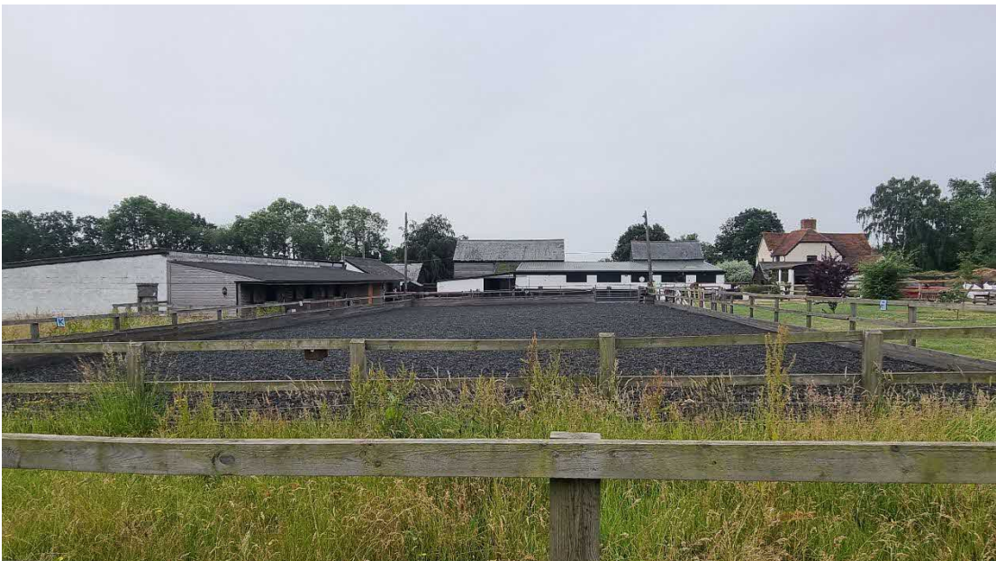
Fig.2: View of Gods Farm looking south, proposal buildings to left, 19 th century barns with Class Q to centre, and listed farmhouse to right.
