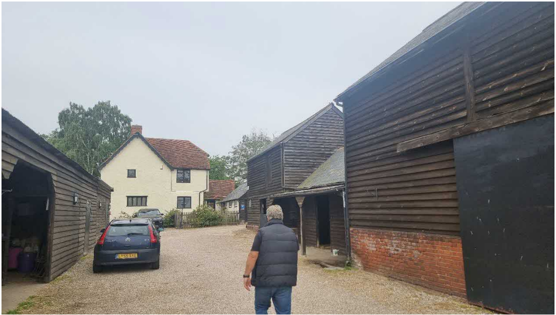
Fig.3: Looking west towards listed farmhouse and 19 th century barns, Harts Lane to left behind the modern stable.
