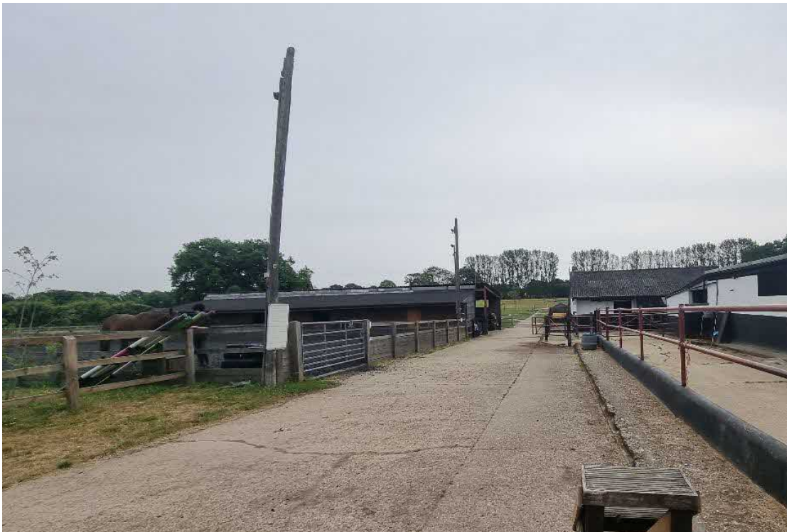
Fig.6: Looking east along from the rear of the 19 th century barns towards the calving building (left) and milking parlour (right, end).
