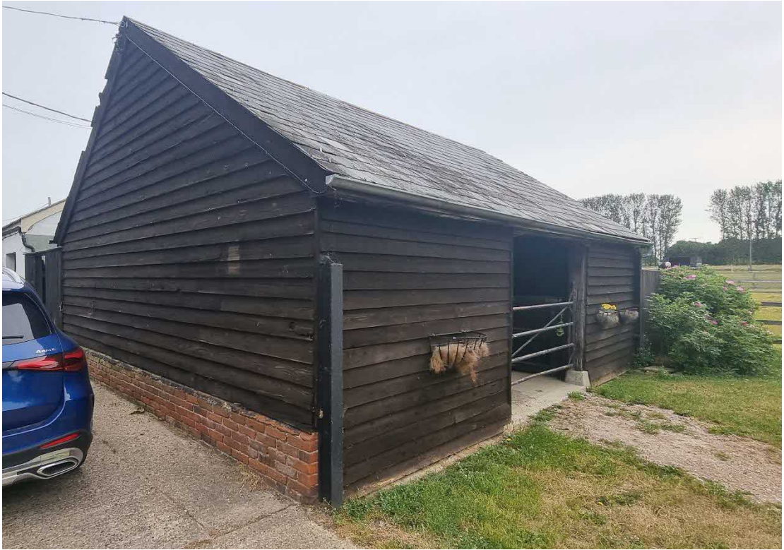
Fig.5: The small weatherboard outbuilding which stands between the modern buildings forming the proposal and the historic farmyard.
