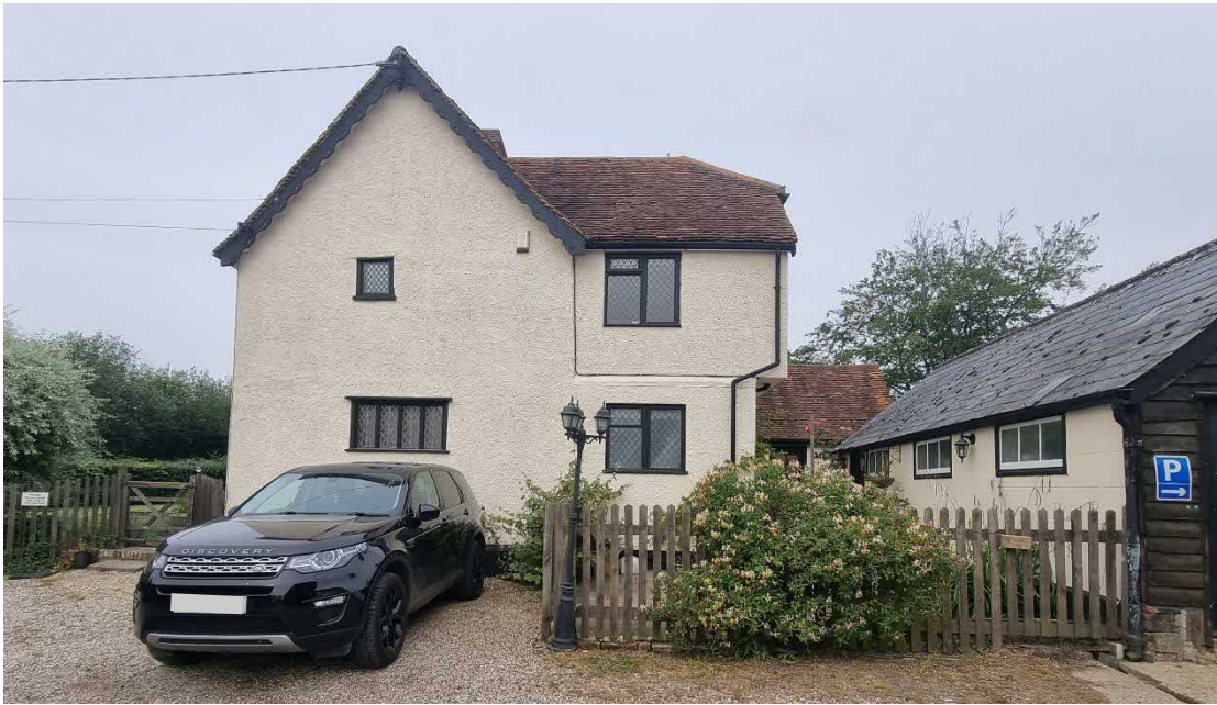
Fig.11: East elevation of the Farmhouse with 21 st century half-hipped first floor addition.
