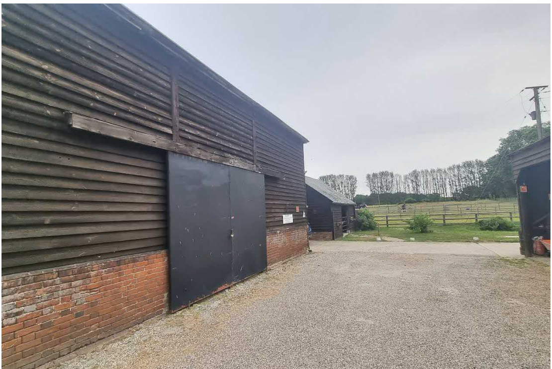
Fig.4: 19 th century barn to left with a smaller timber outbuilding beyond.
