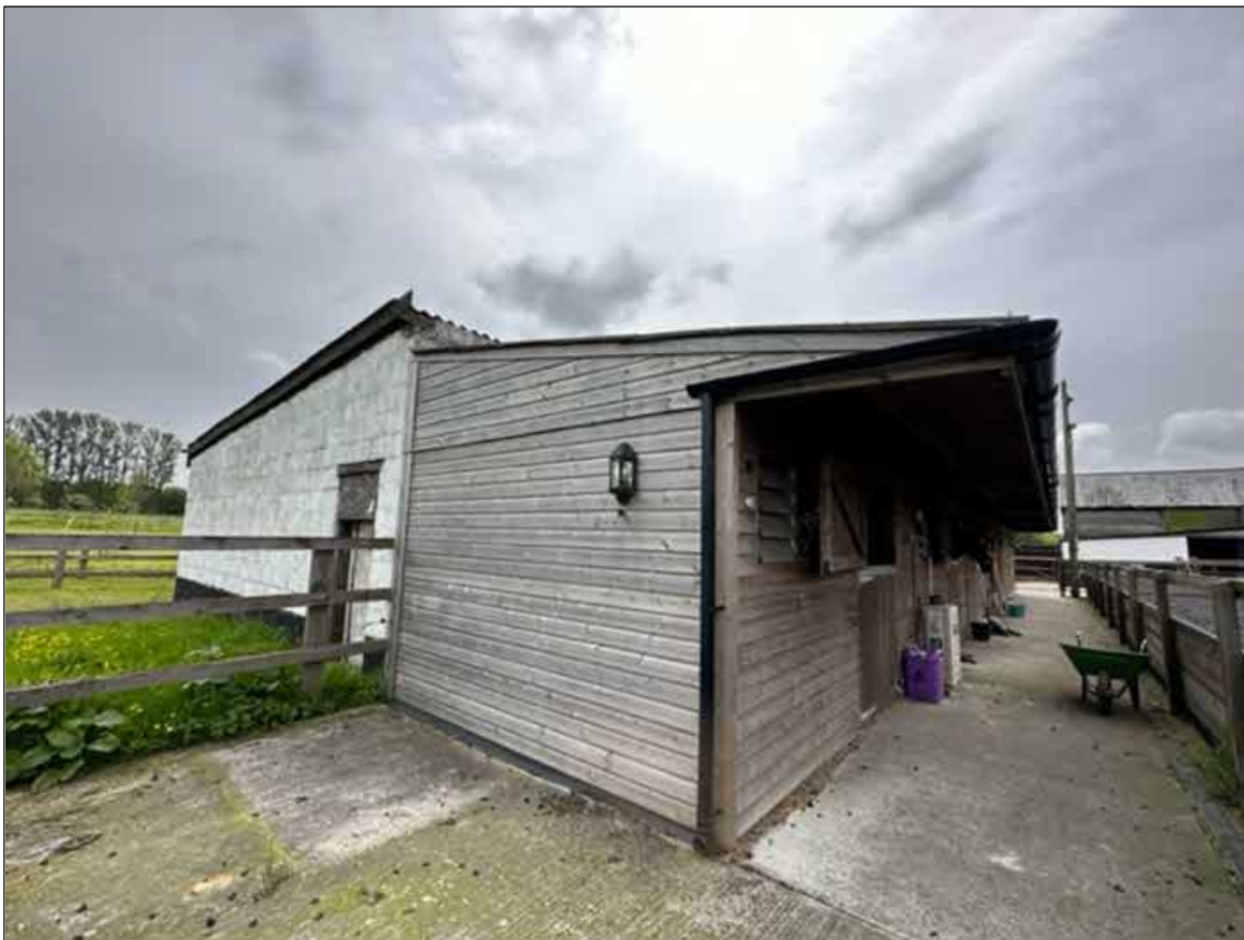
f) Building 3: Northern aspect and adjoining modern stable block.
