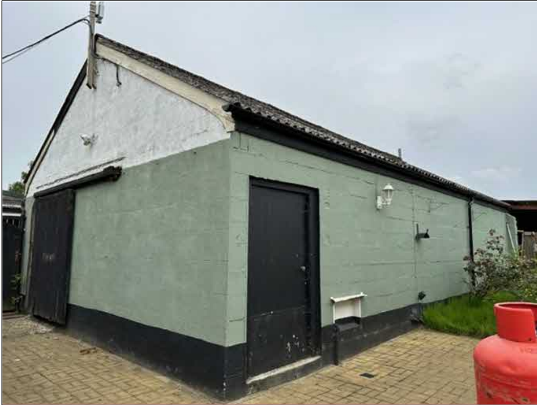
c) Building 2: Southern/western aspect. Fascias/walls are well-sealed.
