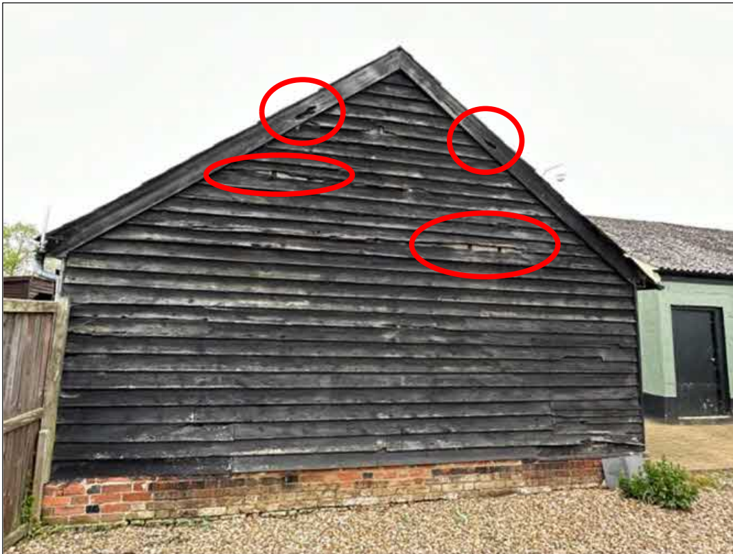
a) Building 1: Various crevices/ingress opportunities on eastern aspect circled.
