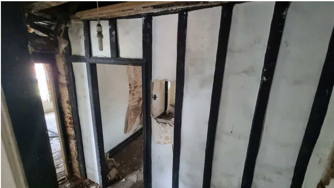
Fig.14: Timber stud wall to first floor.
