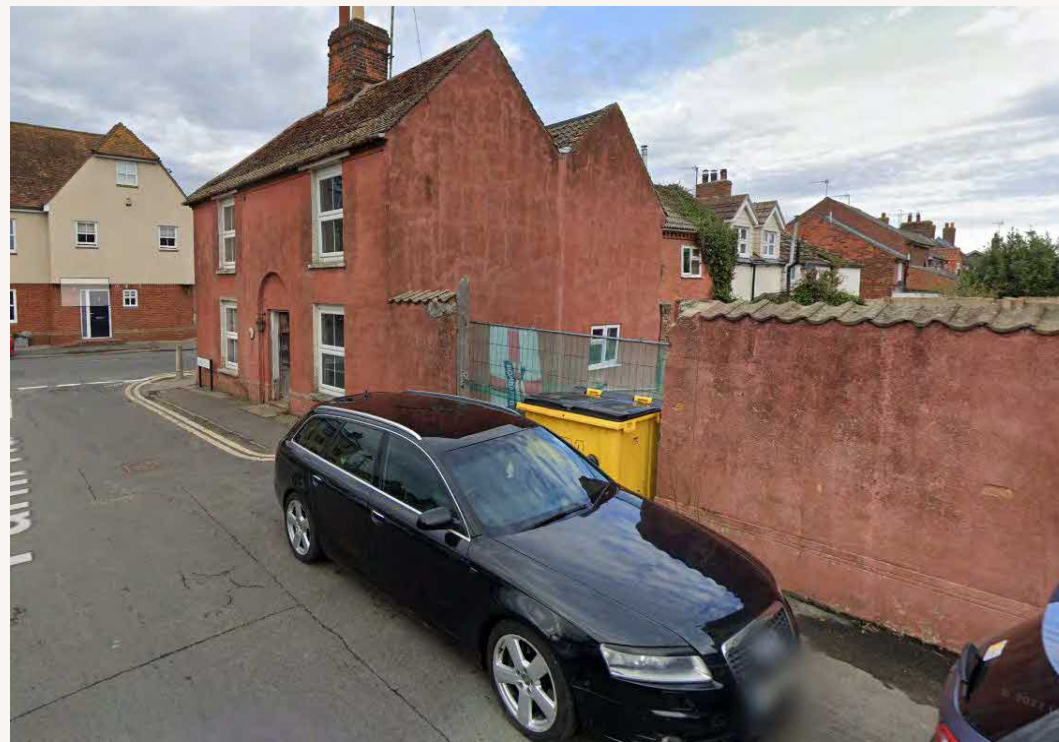
Fig 01 Street View A of site as existing
