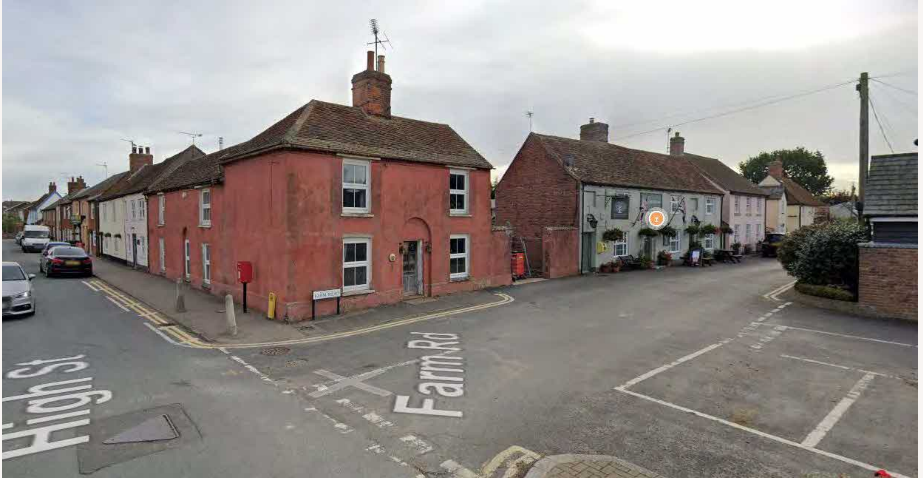
Fig 00. Street view of existing building
