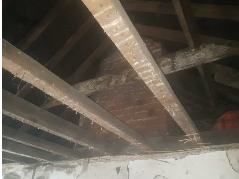
Photograph 11 A Showing roof over Bedroom 3 & high level collar tie.
