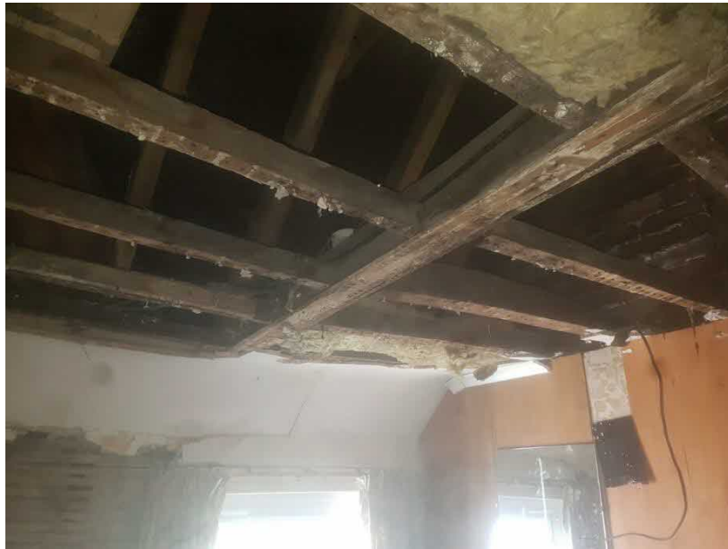
Photograph 19 Showing ceiling structure above bathroom.
