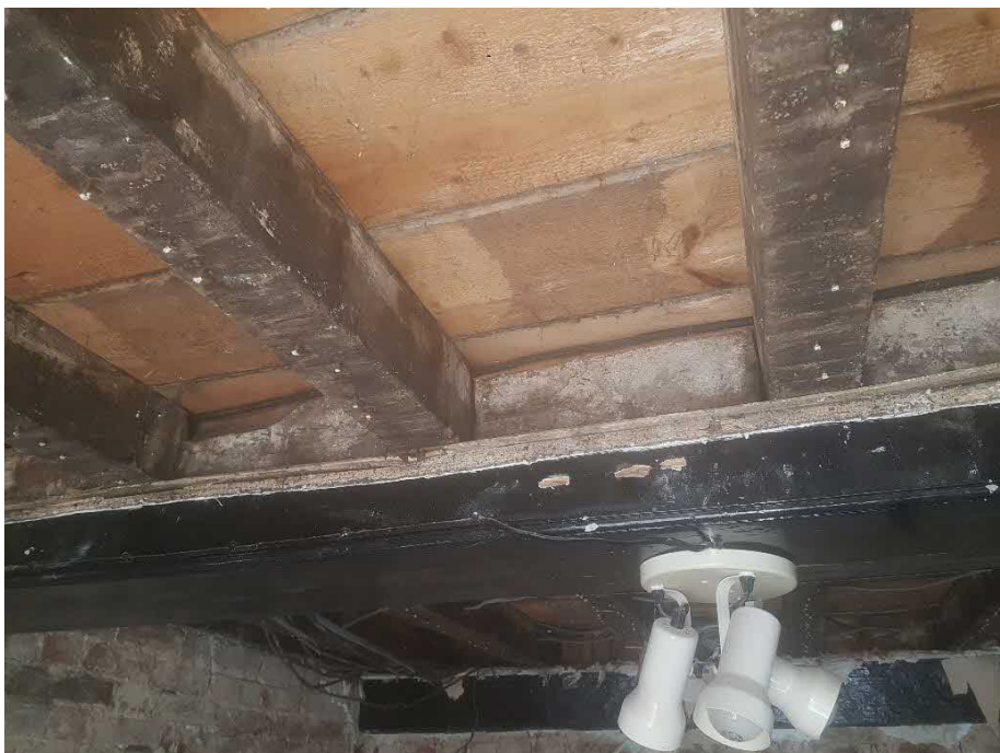
Photograph 29 Showing floor joists and central beam.
