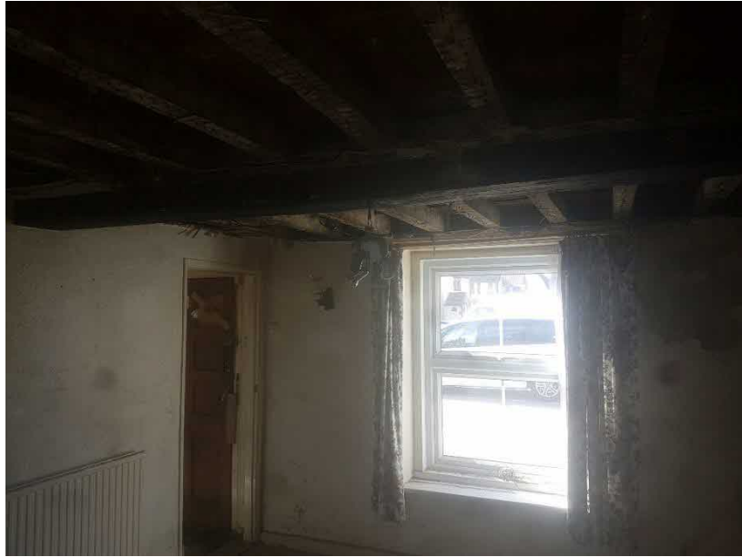
Photograph 21 A Showing lintel over front window in sitting room.
