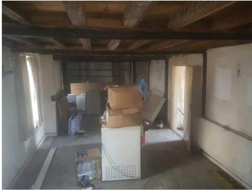
Photograph 23 Showing floor joists and timber beams over living room.
