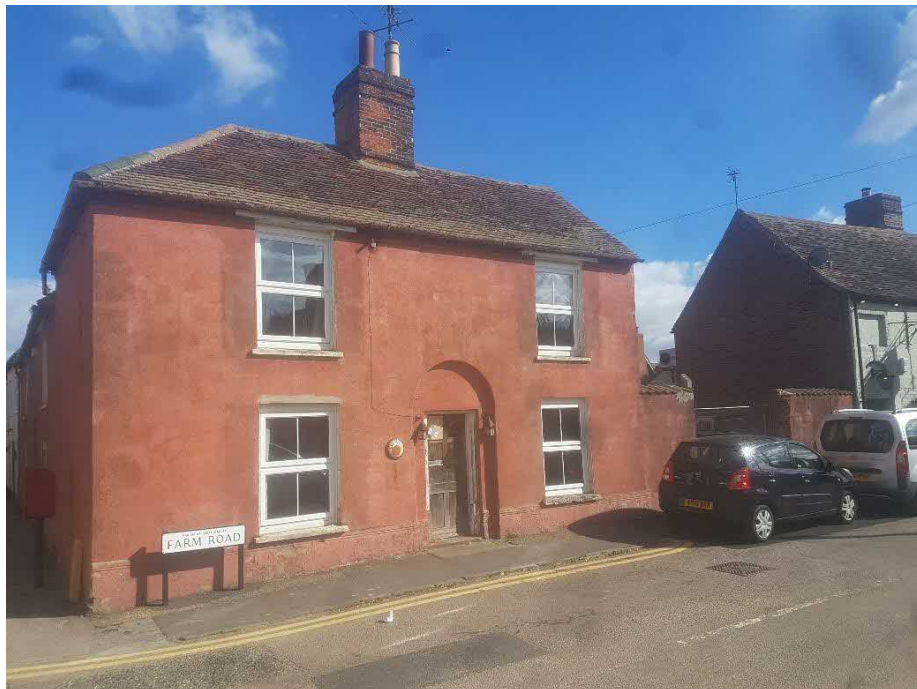
Photograph 1 Showing front (south westerly facing) elevation.
