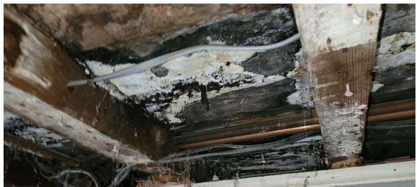
Photograph 18B. Showing view on underside of floor joists and boards.
