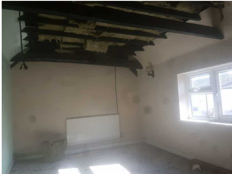
Photograph 10 Showing raised tie roof.
