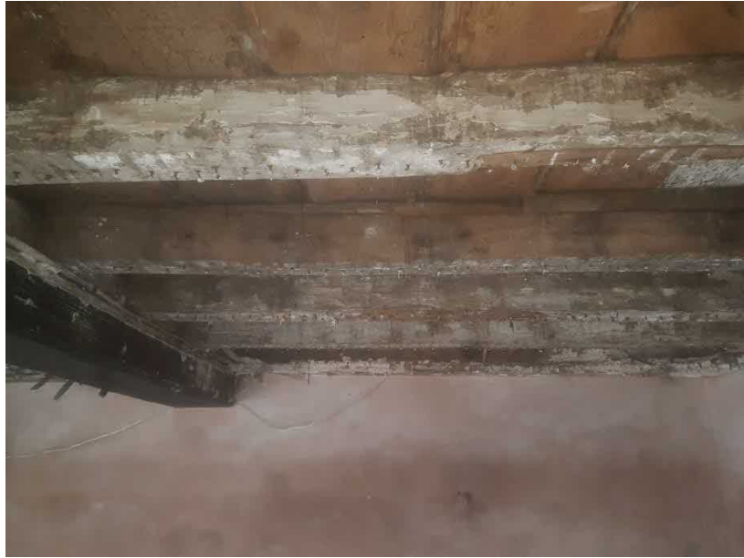
Photograph 20A Showing joists spanning over sitting room.
