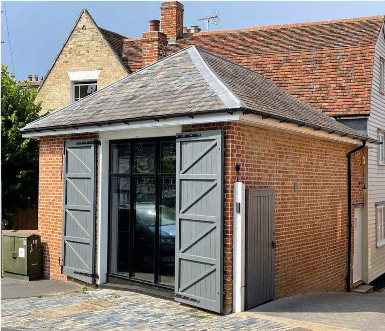
Fig. 6 –Current fenestration at 33 Brook Street.
