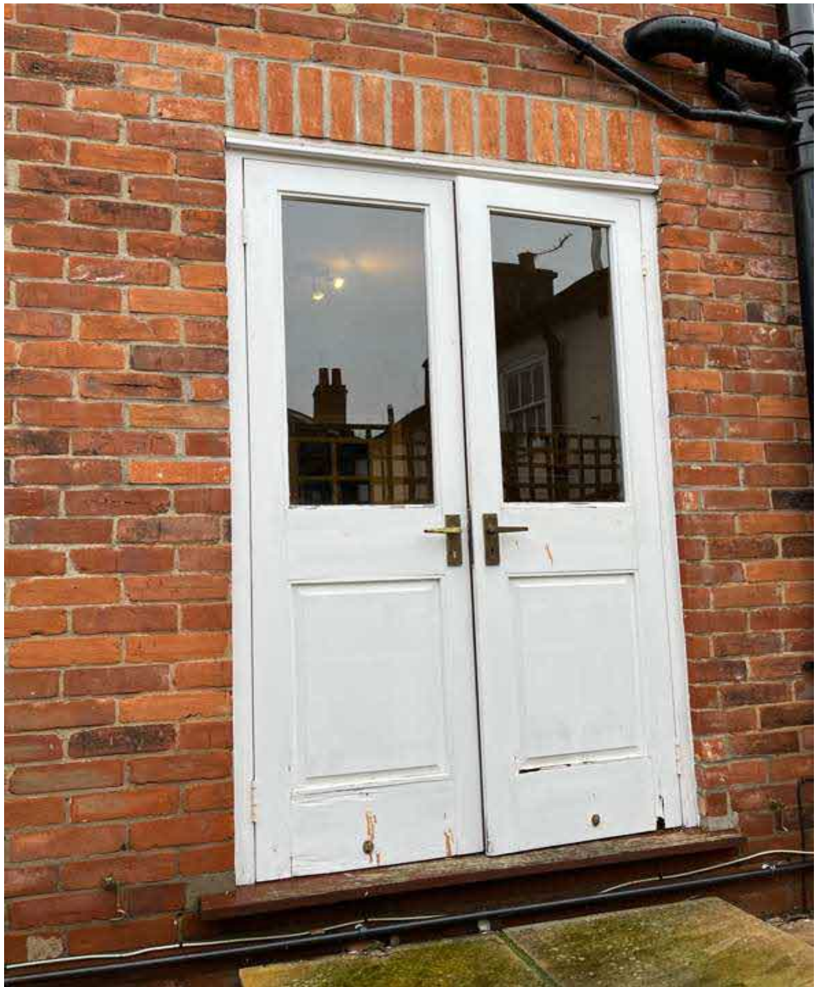
Fig. 1 –External view of existing rear french door.
