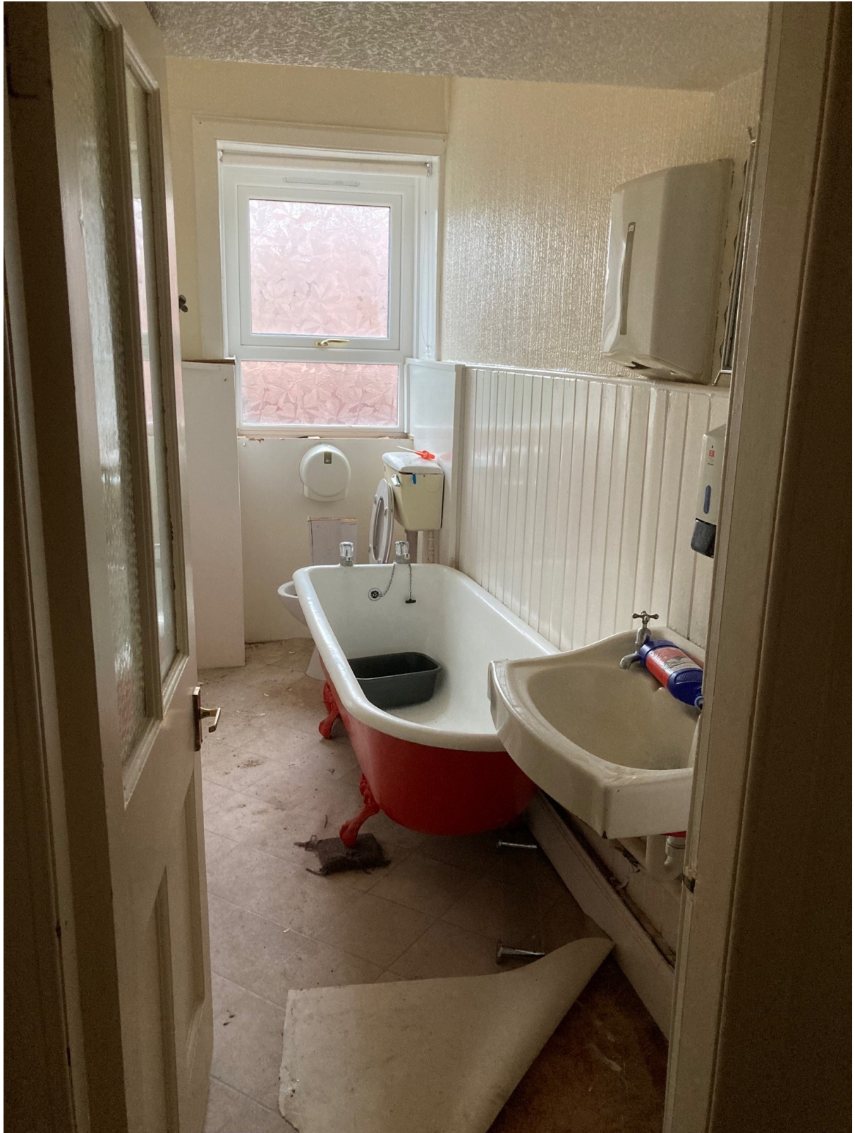
EXISTING GF BATHROOM
