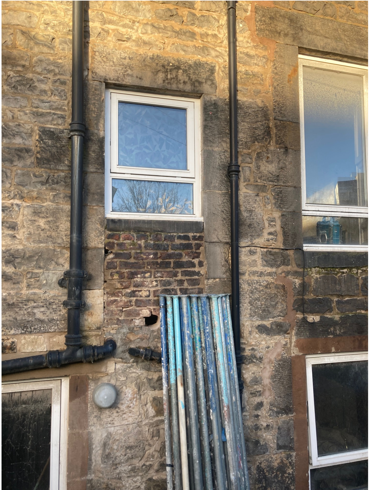
EXISTIONG GF BATHROOM WINDOW SHOWING PREVIOUS DOOR OPENING INFILLED
