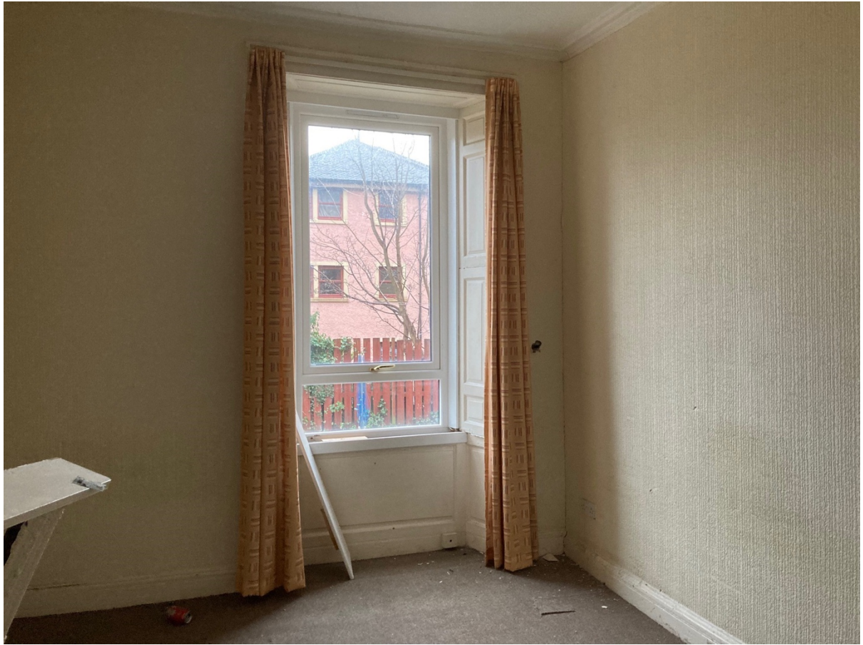
EXISTING REAR ROOM SHOWING EX BATHROOM WALL
