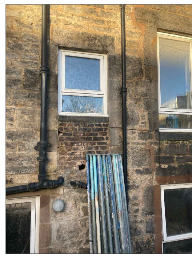
Existing bathroom rear window
