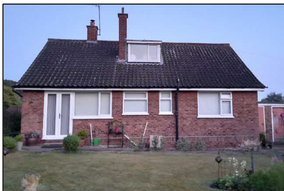
Figure 1: Rear view – eastern aspect
