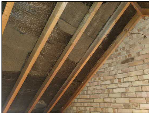
Figure 3: Right hand garage open to roof structure.
