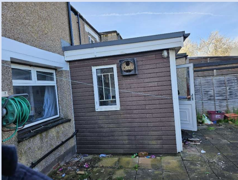
Side view of the existing extension
