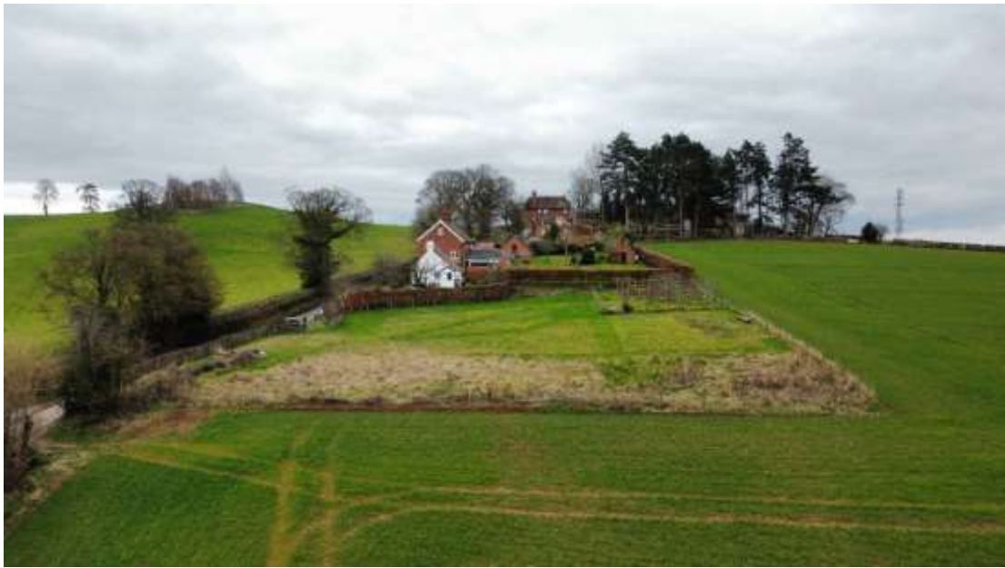
Photo 1 - The Site looking towards the current dwellings of Round Oak Cottage, and Elm Cottage.
