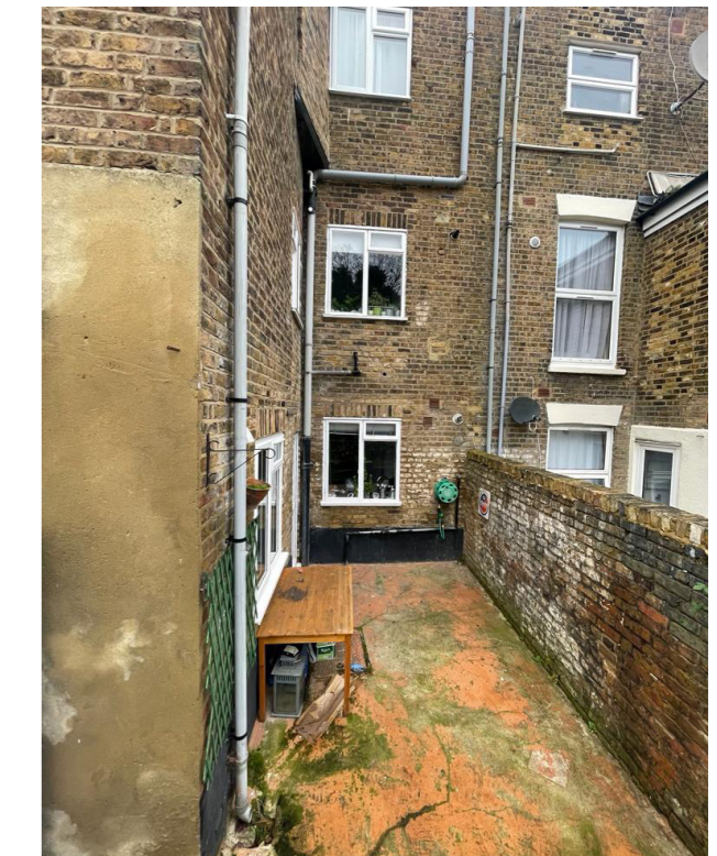
.Existing yellowstock brick facade and concrete slab floor
