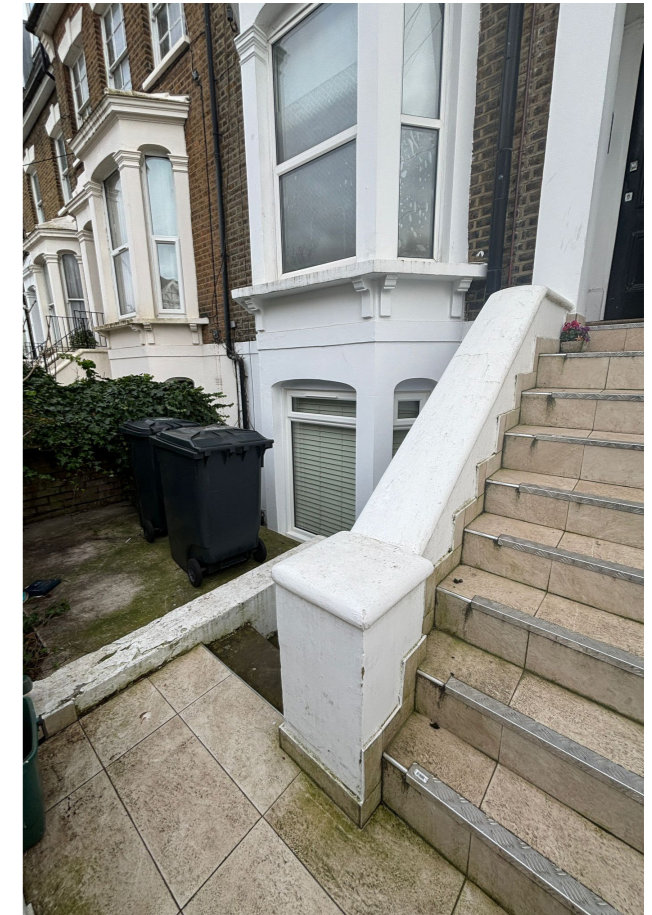
.Common entrance with bin area
