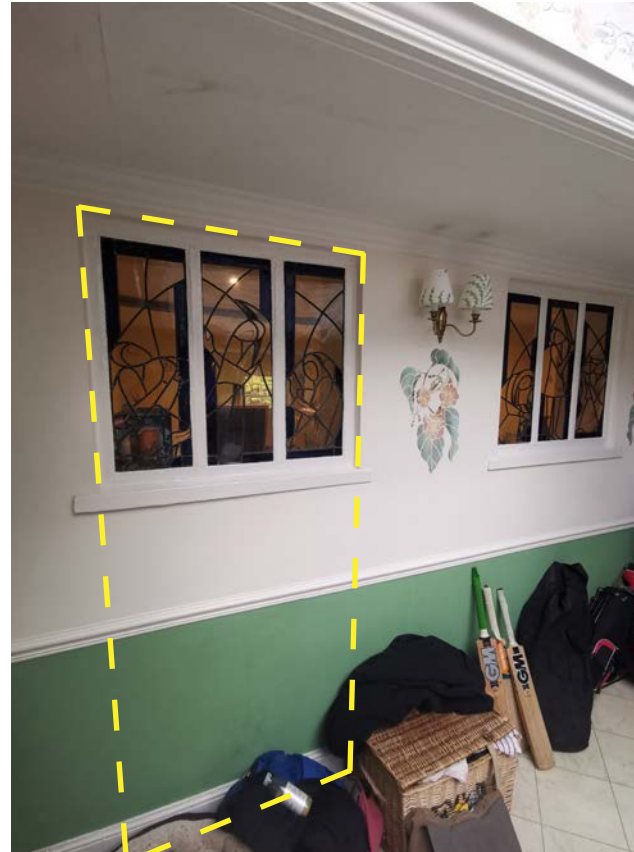
Photograph of the existing window (left) to be opened up to form new doorway into boots room. The window on the right of the photograph will remain.
