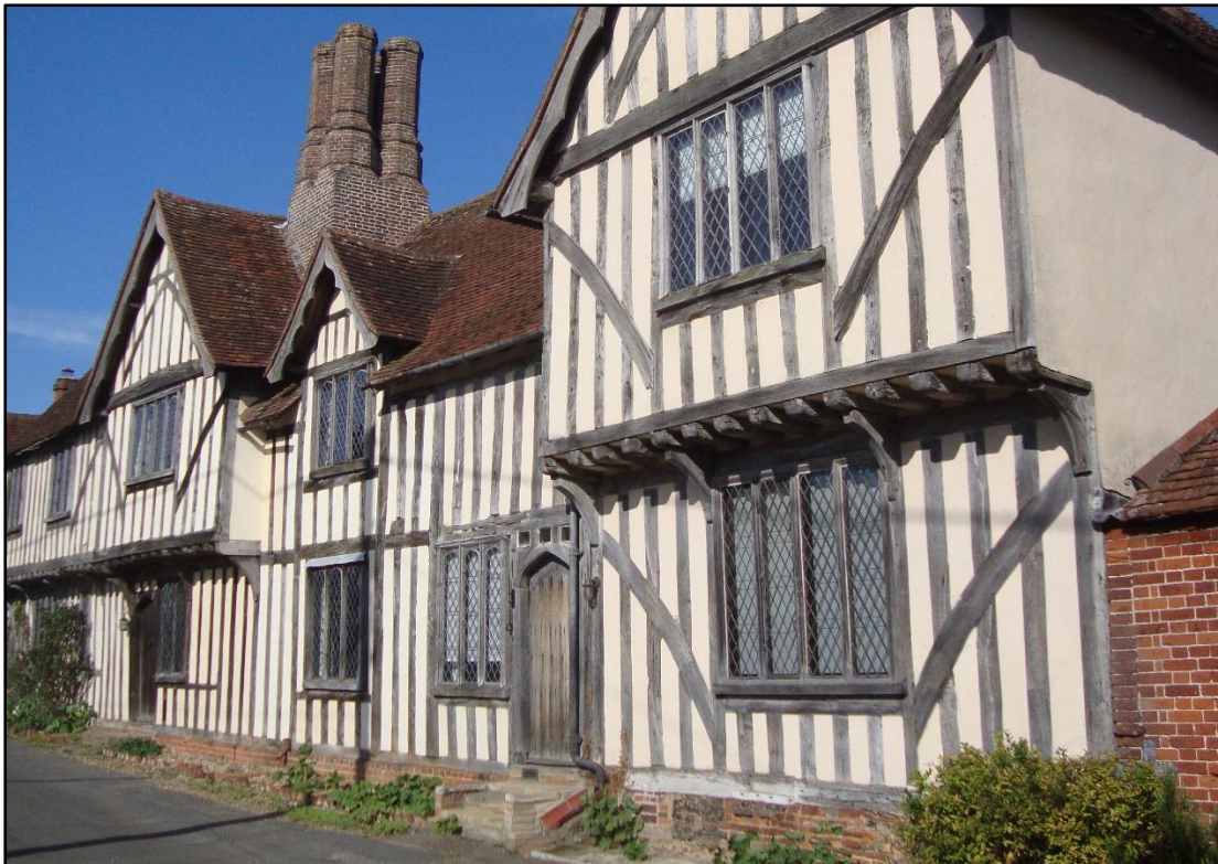
Fig.16 Nos. 3 and 4 Maltings Cottages
