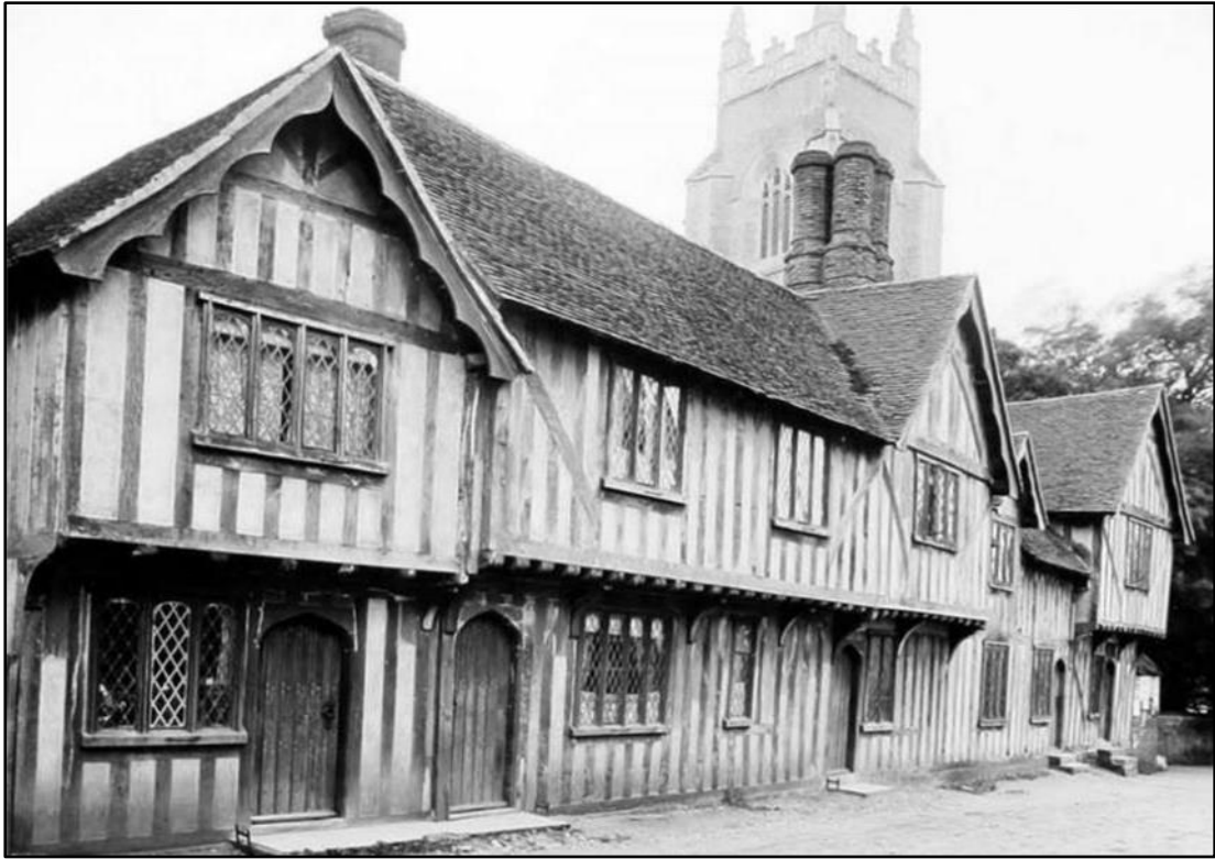
Fig.15 Row of five cottages (photographed early C20)
