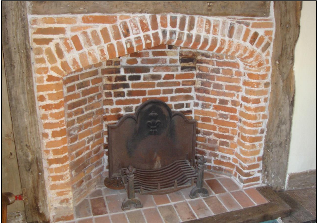
Fig.28 Fireplace in main bedroom
