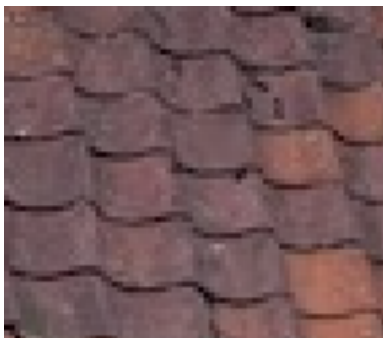
Existing clay pantiles.
