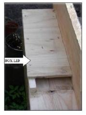
**Integrated roost feature** under barge boards at gable end.
