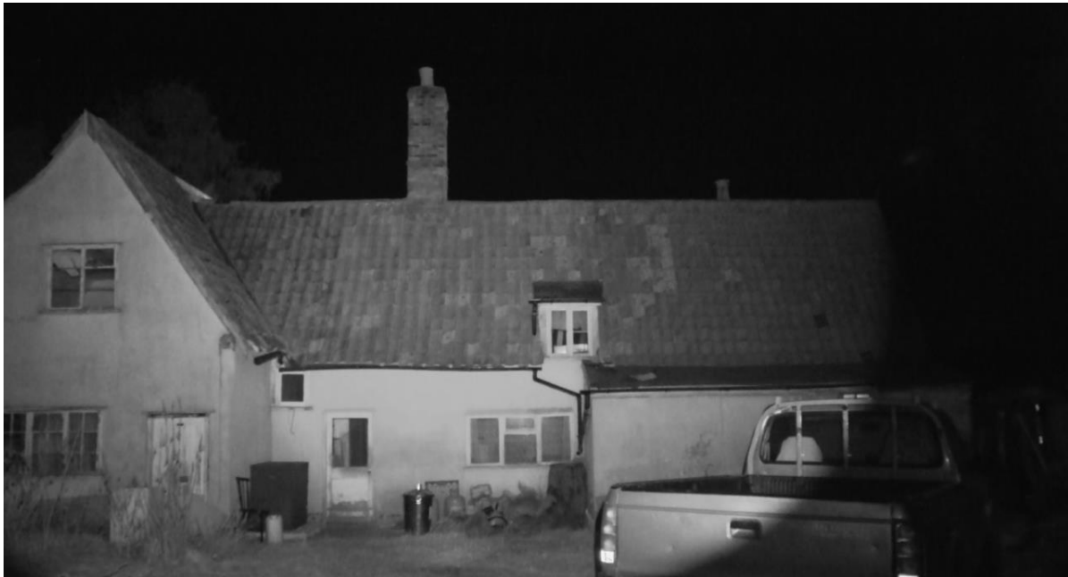
Plate 3.4: Canon XA11 with Nightfox XB5 and 12-Led 90°Wide Angle IR Illuminator – south-western elevation of Cottage – 03.09.23.
